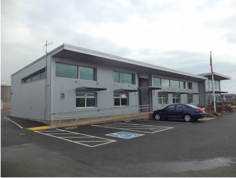
Building B & C (Divis & Lockers)
