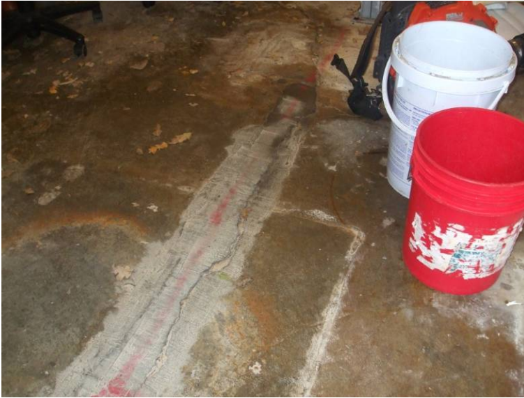
Pool Pump Building
