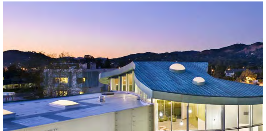
Connection Center View
