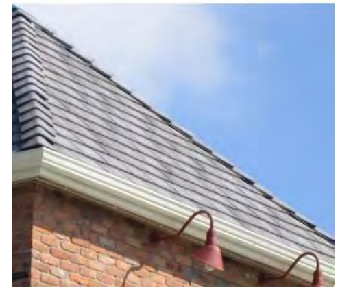
COMPOSITE SHINGLE ROOF
