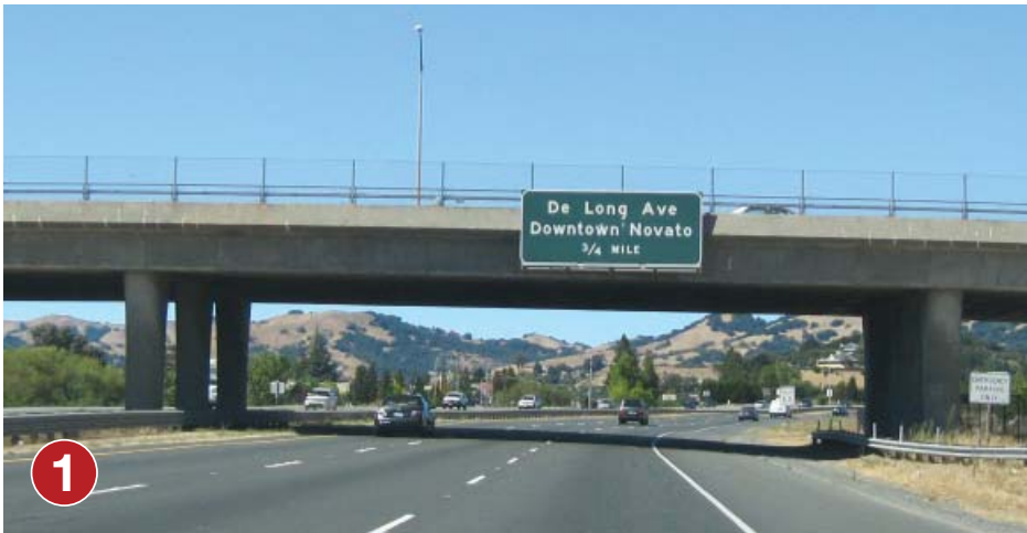
Rowland Boulevard overpass Sign location OK.
