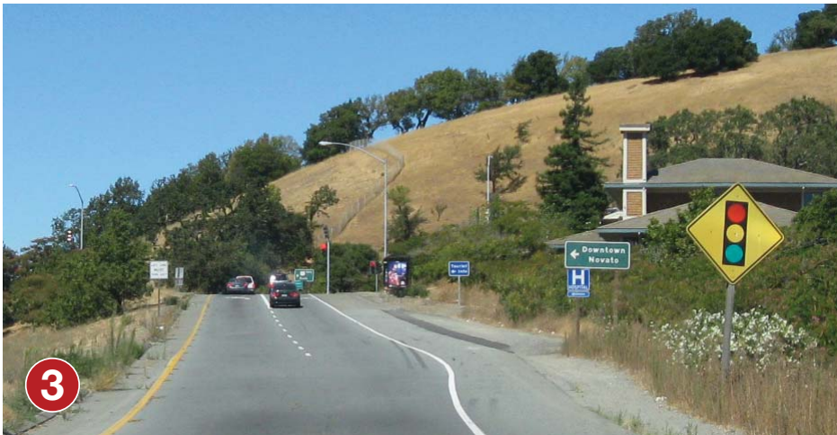
De Long Avenue exit ramp Sign locations OK. Consistent message.
