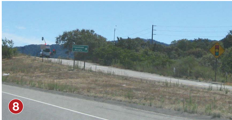
8 De Long Avenue exit ramp Sign location OK. Consistent message.
