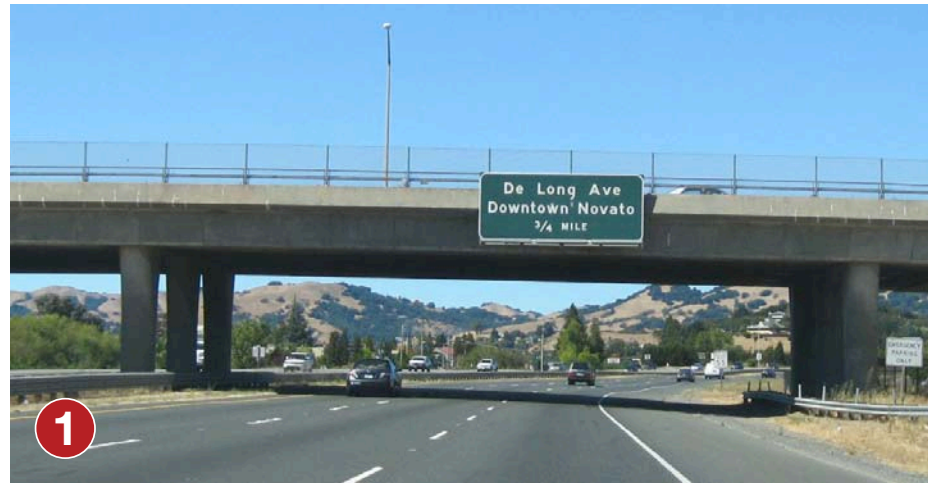
Rowland Boulevard overpass Sign location OK.
