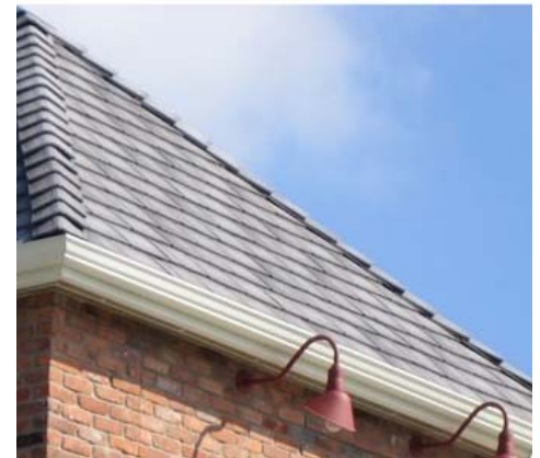
COMPOSITE SHINGLE ROOF
