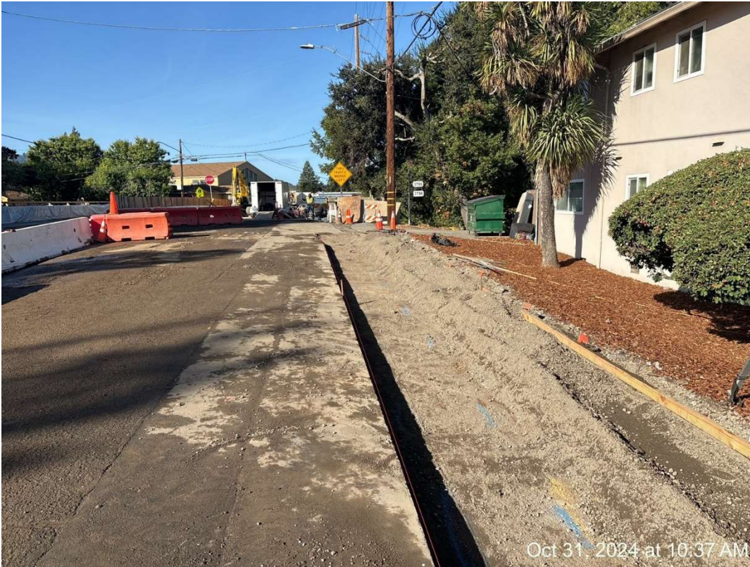
Figure 26 – Northside Sidewalk Demolished.
