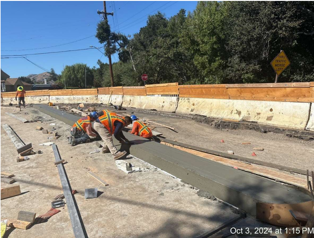
Figure 1 – Pouring Bridge Median Curb.
