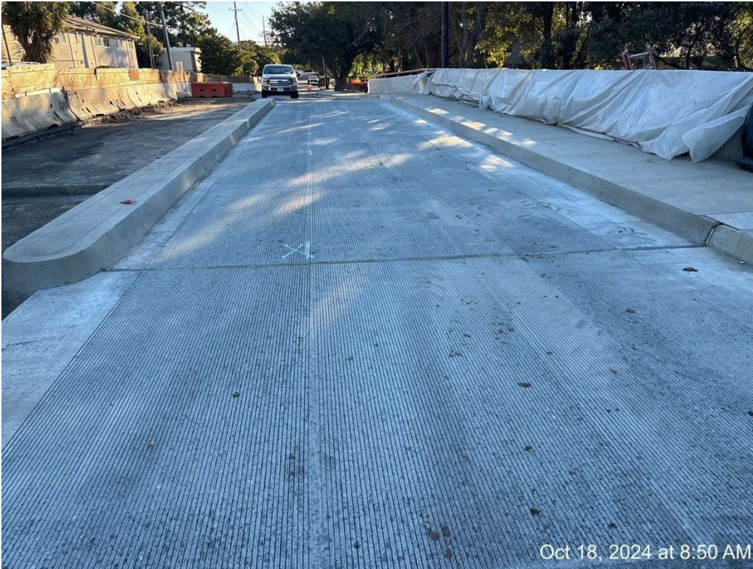
Figure 20 – Completed Grooved Bridge.
