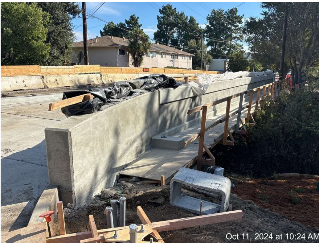
Figure 2 – Class 1 Finish on Type 732 SW Barrier.
