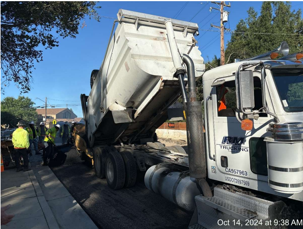
Figure 12 – HMA Paving.
