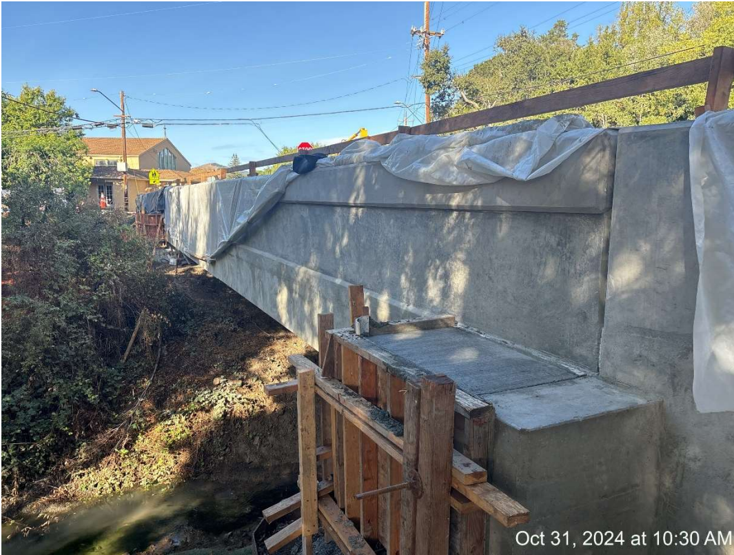
Figure 22 – Completed Exterior Shear Keys.
