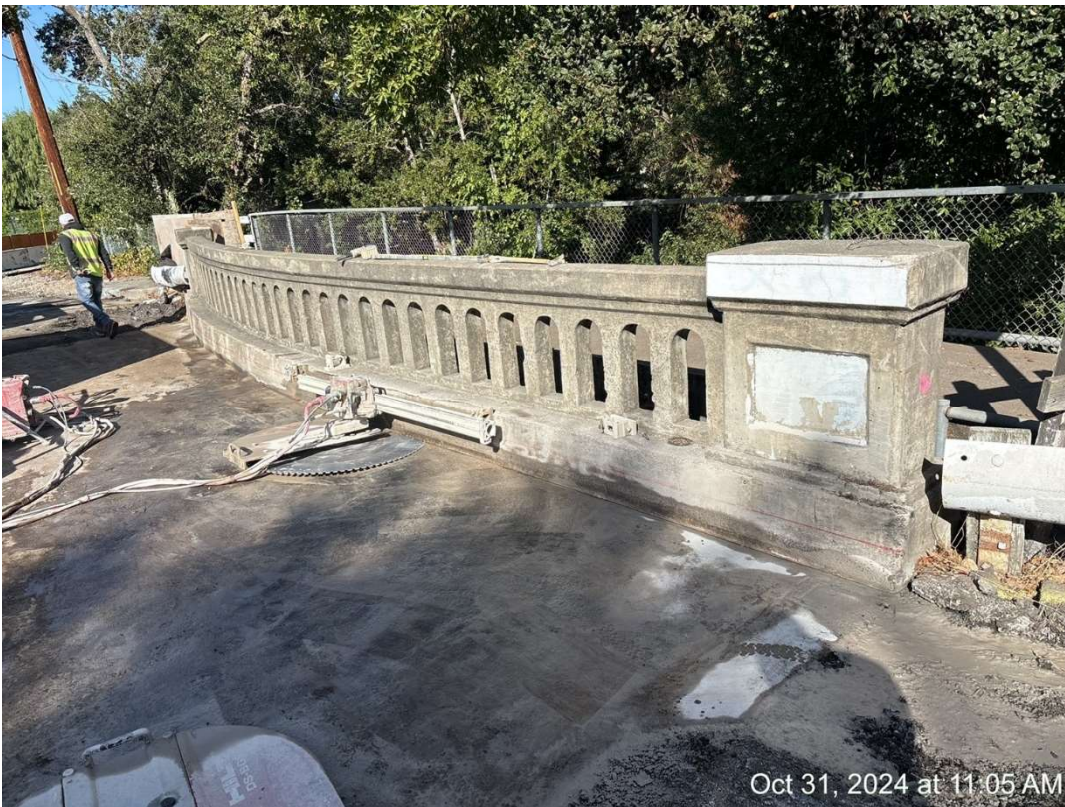
Figure 27 – Sawcutting Northside Barrier.
