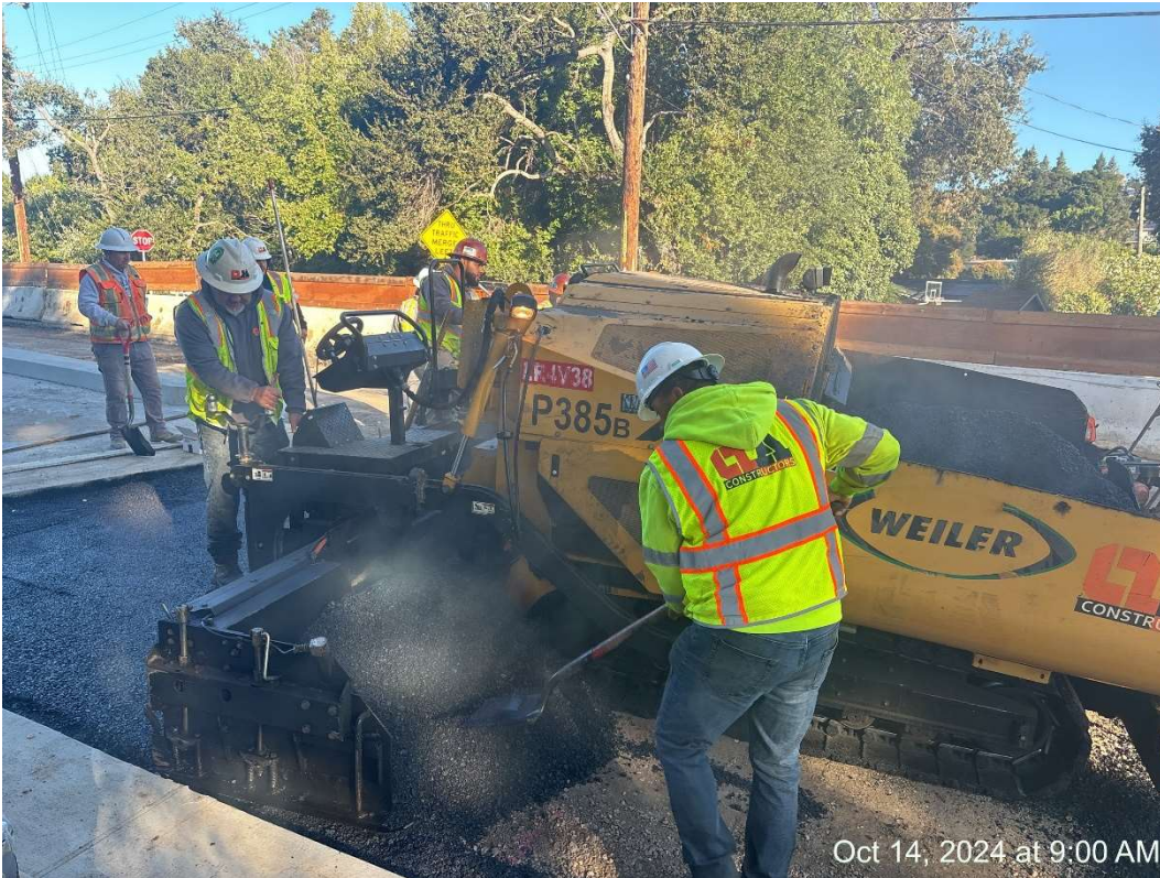
Figure 10 – HMA Paving.
