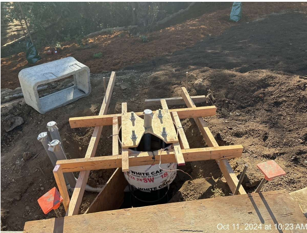
Figure 6 – Forming Light pole foundation.
