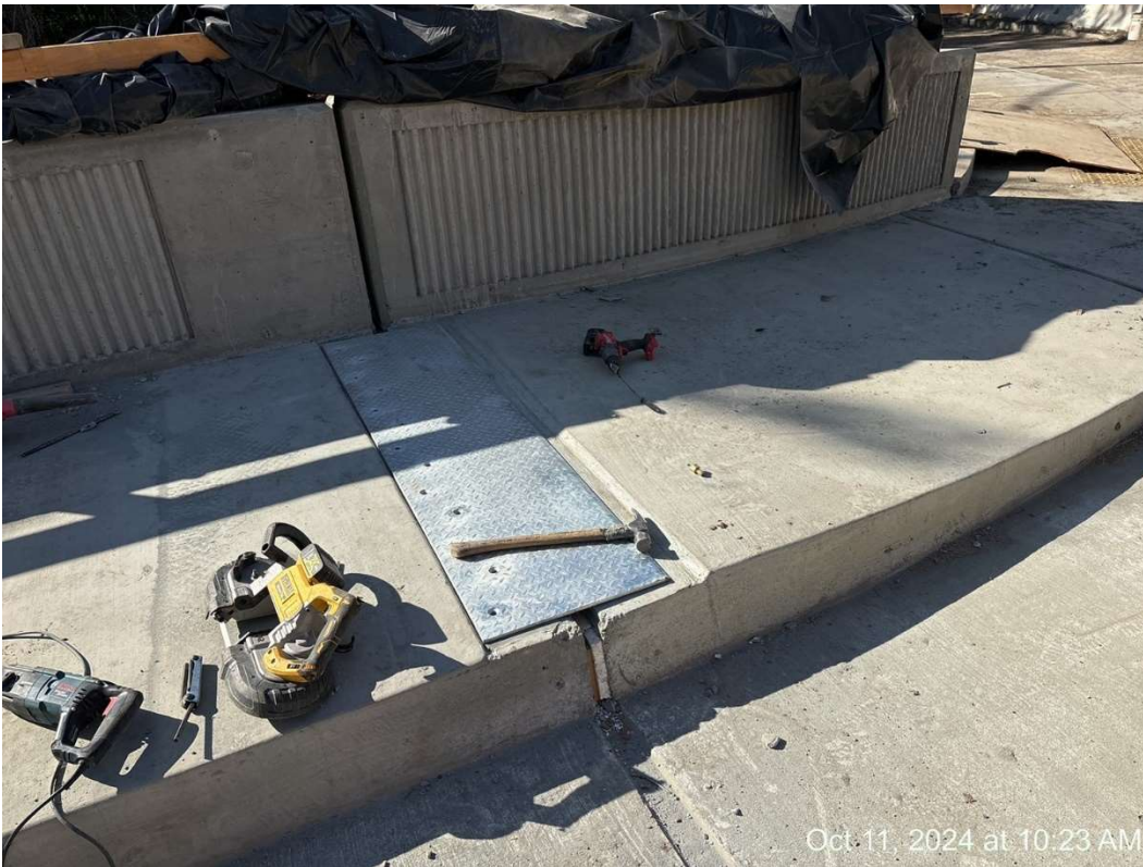
Figure 5 – Installing Sidewalk Joint Cover Plate.
