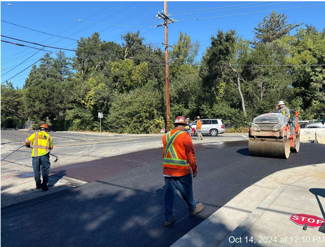
Figure 14 – Paving the West Side of Stage 4.
