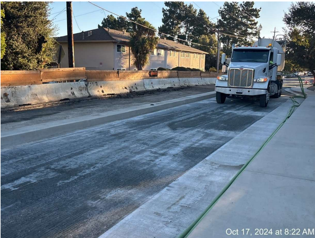
Figure 17 – Grinding the Bridge (ABSL).
