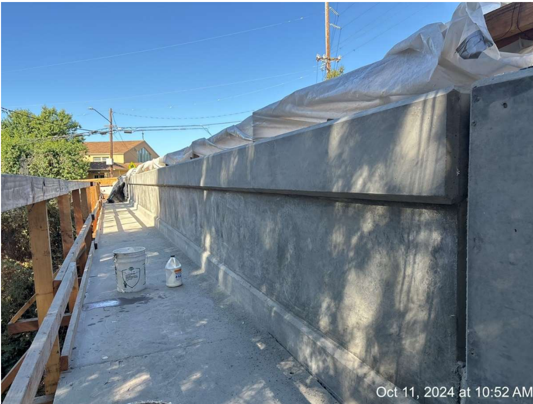
Figure 3 – Class 1 Finish on Type 732 SW Barrier.
