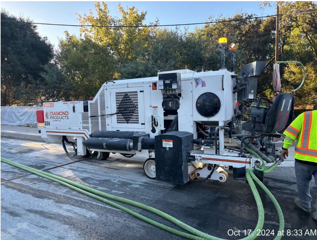
Figure 18 – Grinding the Bridge (ABSL).
