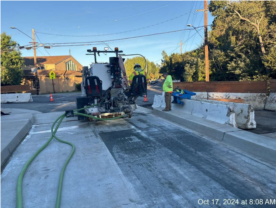
Figure 16 – Grinding the Bridge (ABSL).
