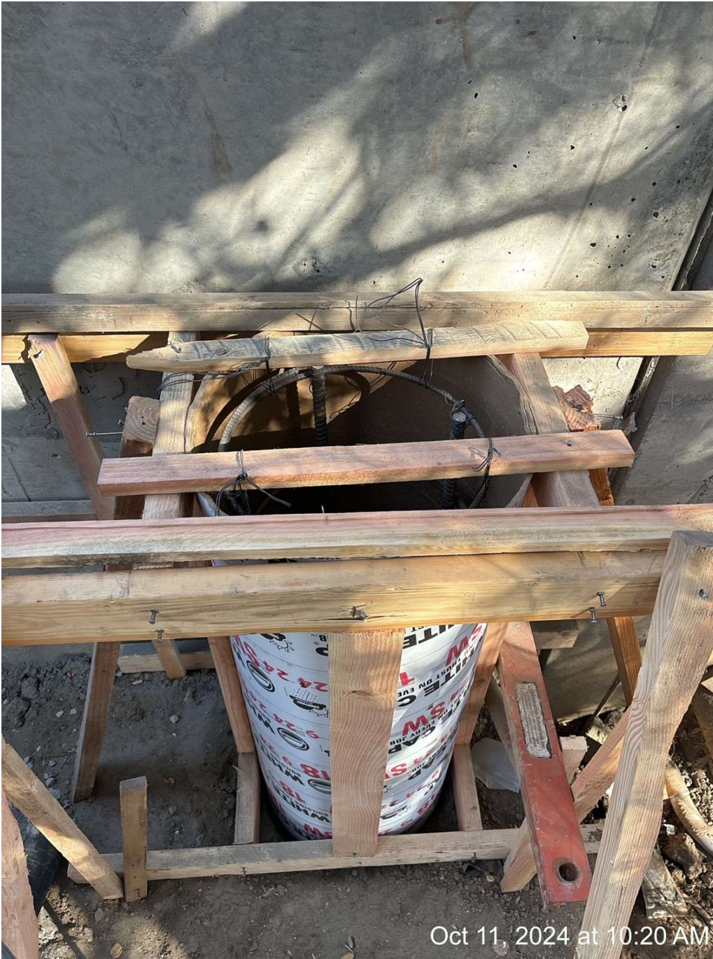
Figure 7 – Forming Light pole foundation.
