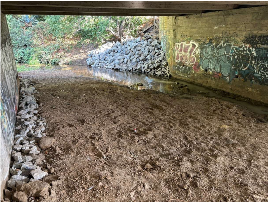
Figure 35 – Creek Restoration, RSP, and Planting.
