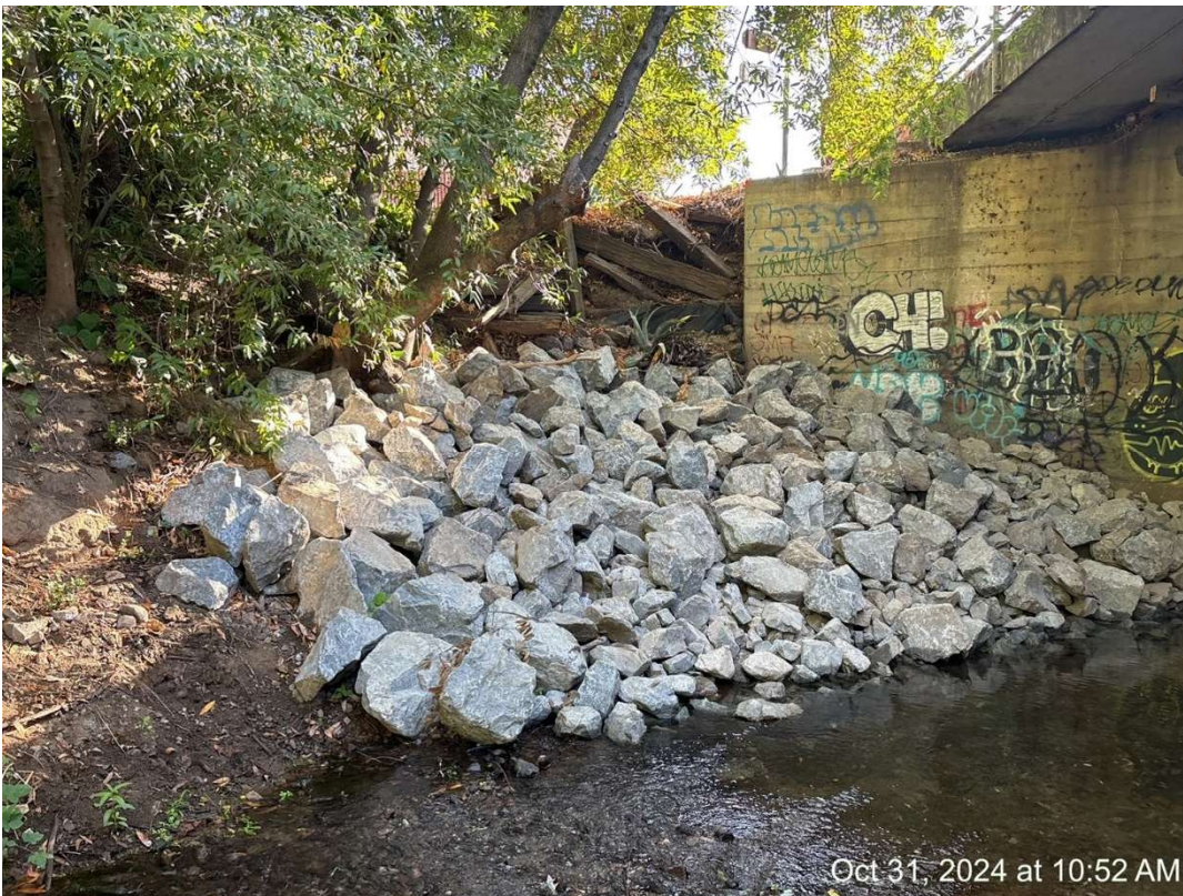
Figure 37 – Creek Restoration, RSP, and Planting.
