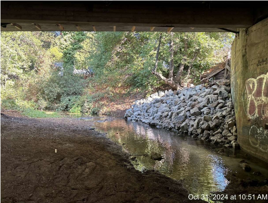
Figure 36 – Creek Restoration, RSP, and Planting.
