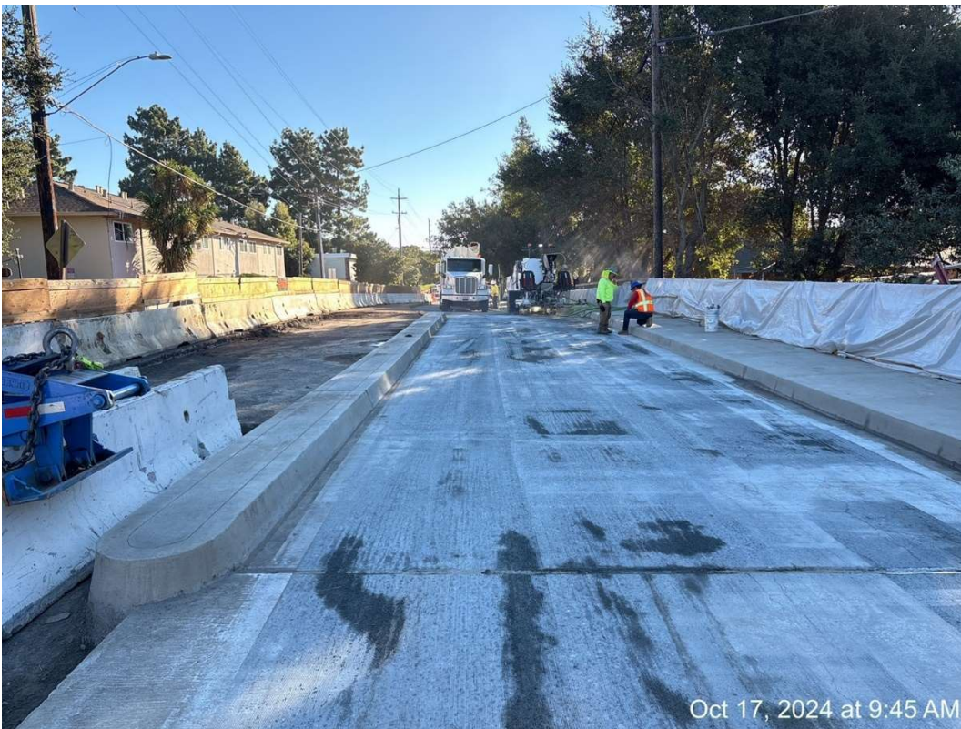
Figure 19 – Grinding within specifications.
