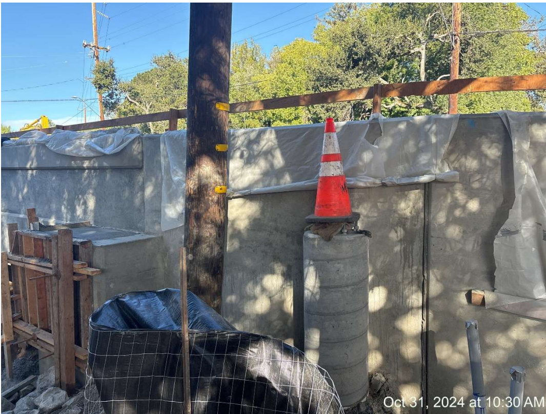
Figure 21 – Poured Lightpole Foundation.
