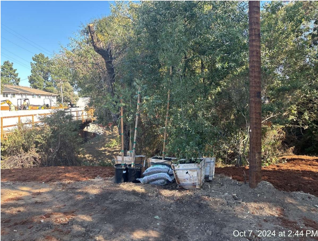
Figure 8 – Begin Planting and Remediation.
