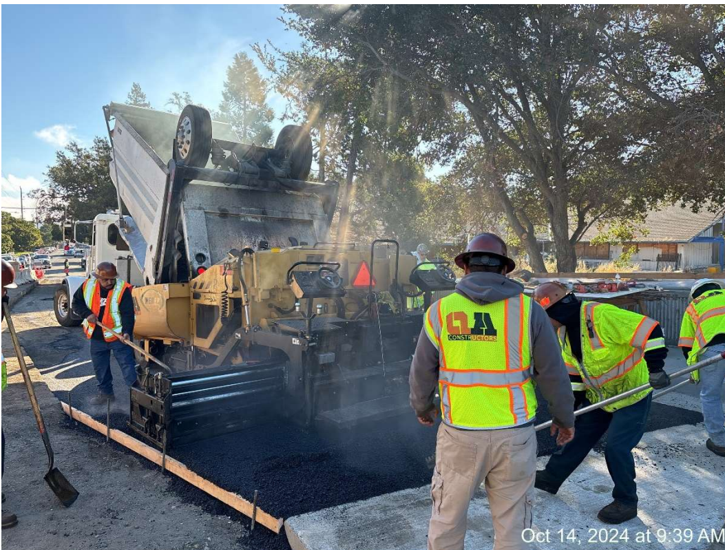
Figure 11 – HMA Paving.
