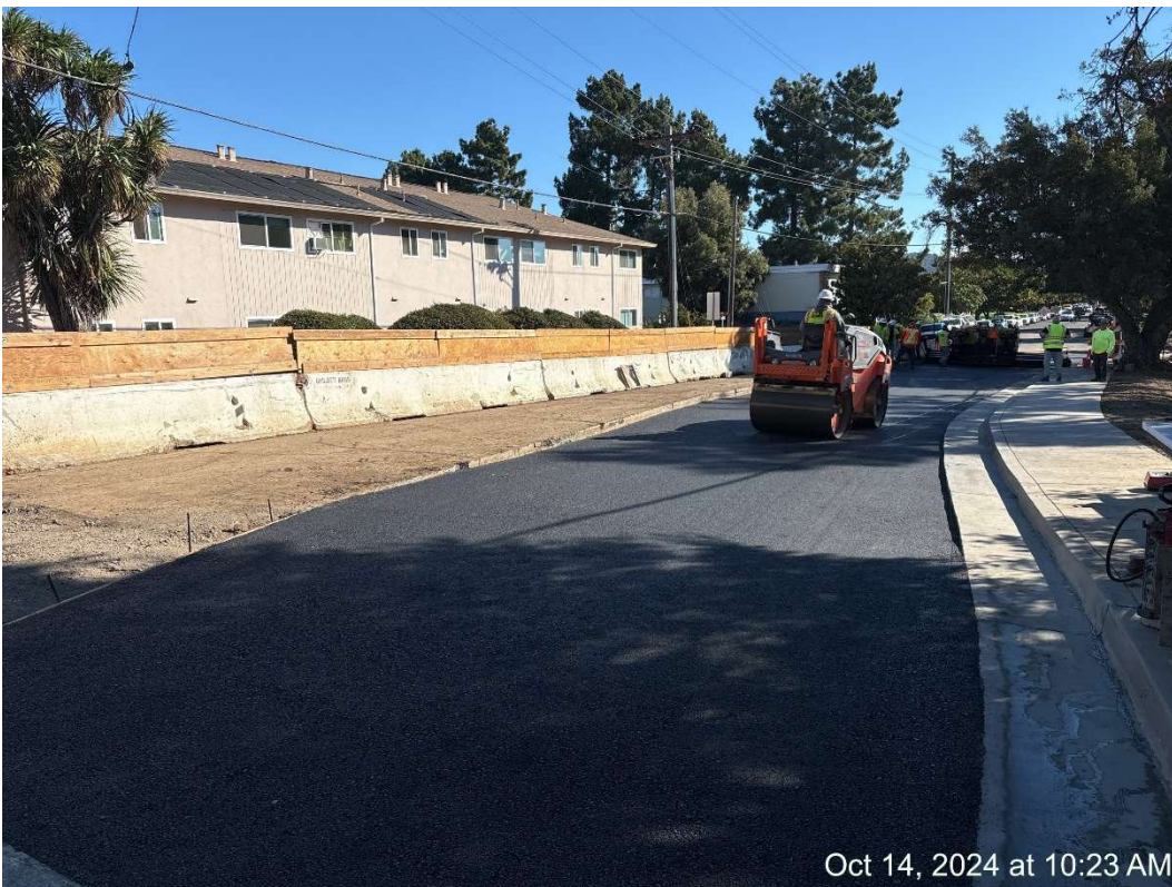
Figure 13 – Breakdown Rolling.
