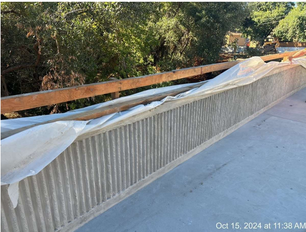
Figure 4 – Interior Formliner Finish – Fractured Fin.
