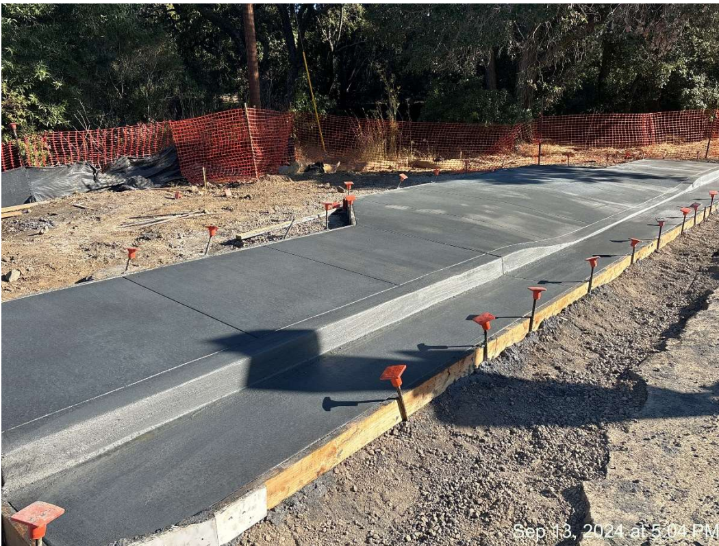
Figure 6 – Poured West Driveway.
