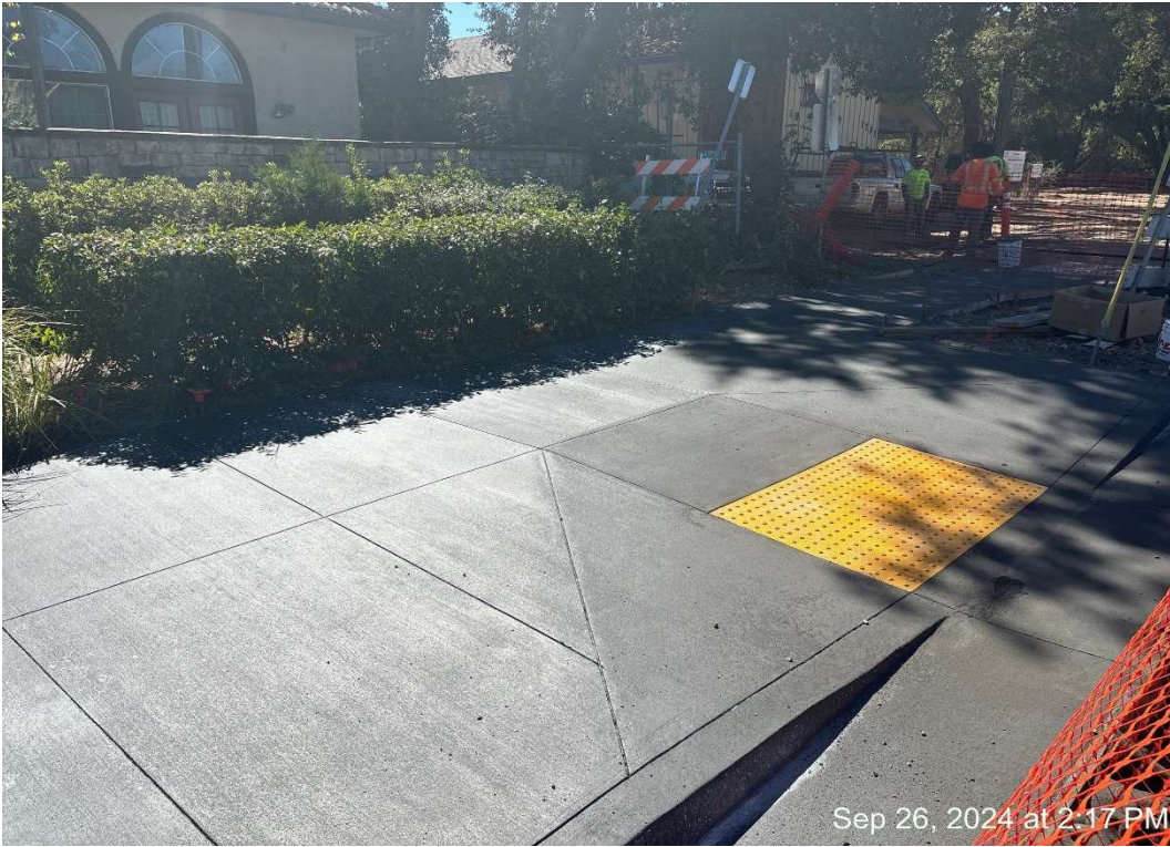
Figure 11 – Completed Type B Ramp at Southeast.
