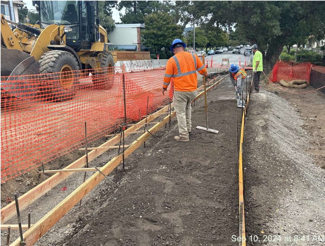
Figure 5 – Forming Curb, Gutter & Sidewalk by Cork Oak.
