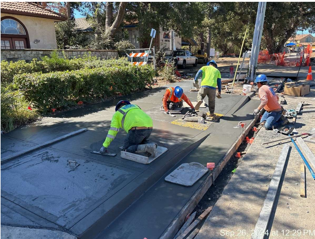
Figure 10 – Pouring Southeast Type B Ramp.
