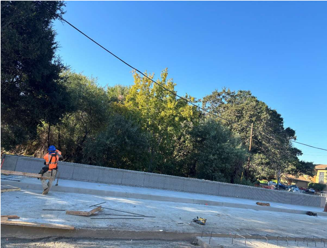
Figure 15 – Bridge Barrier Poured.
