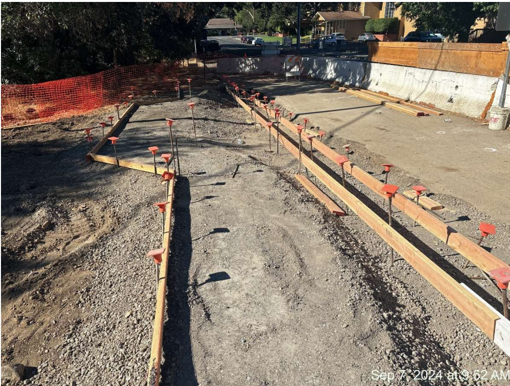
Figure 4 – Forming West Driveway.
