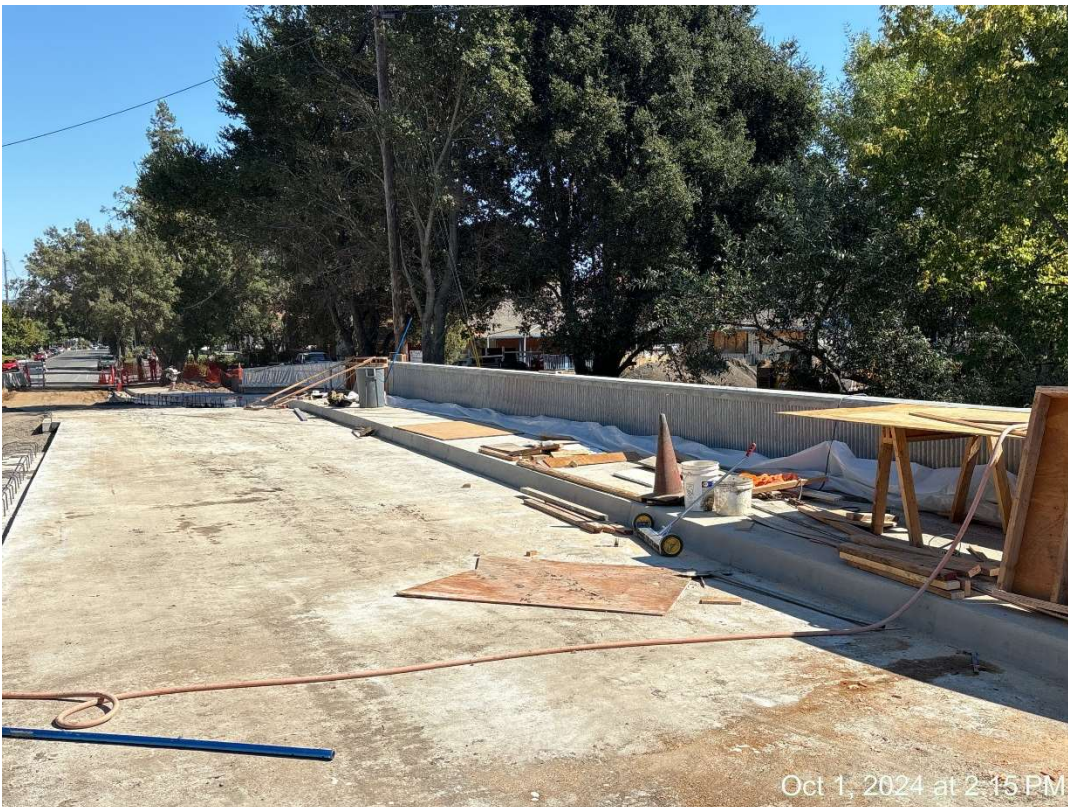
Figure 18 – Barrier complete.
