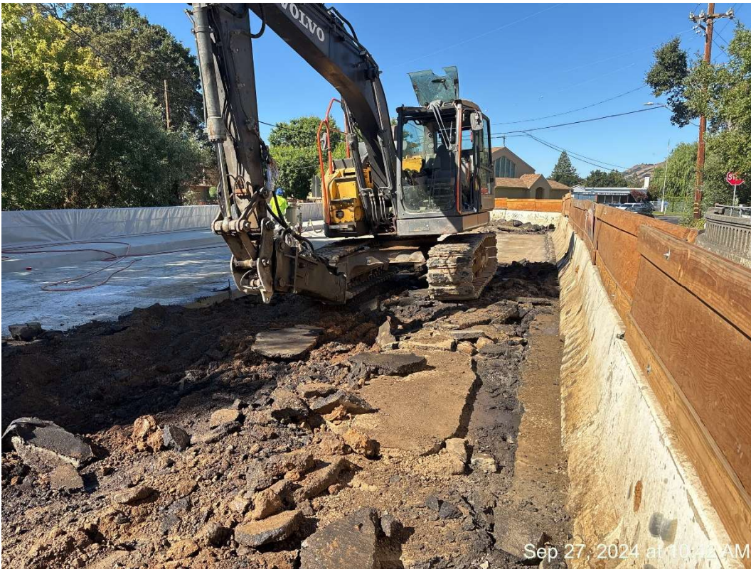
Figure 19 – Obliterating existing Pavement.
