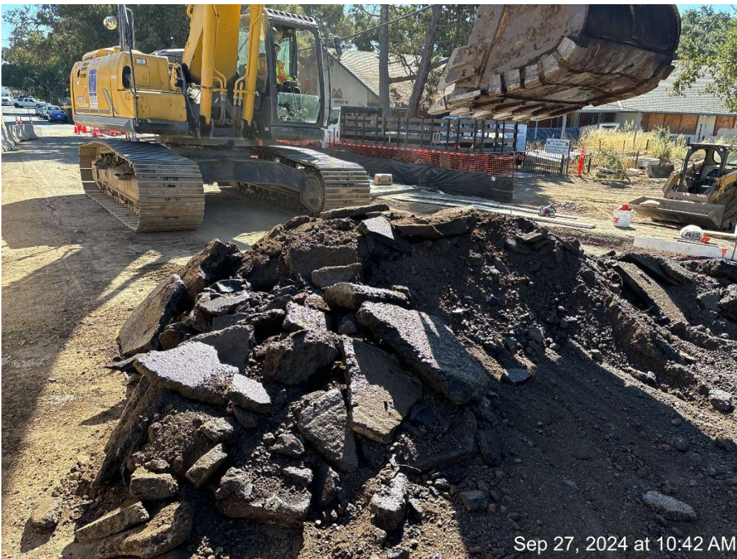
Figure 20 – Obliterating existing Pavement.
