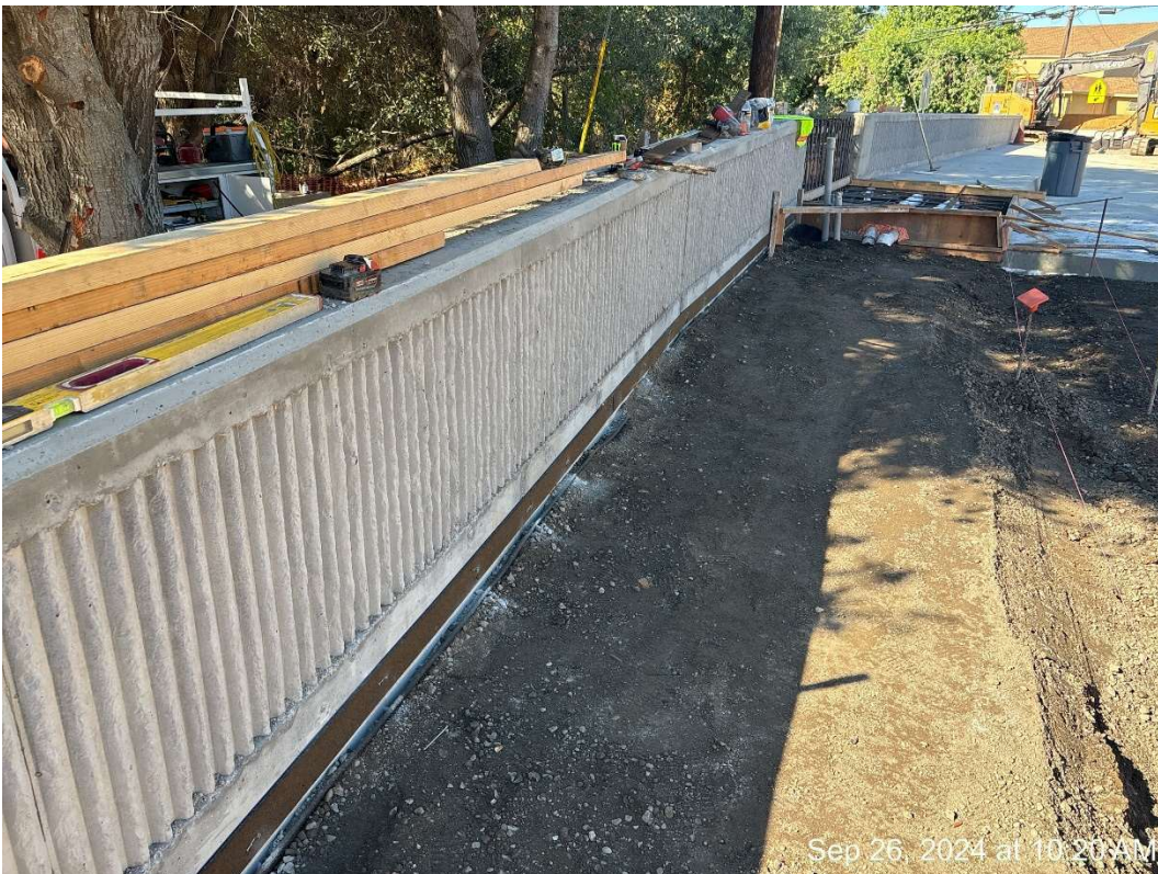
Figure 8 – Stripped Retaining wall forms.
