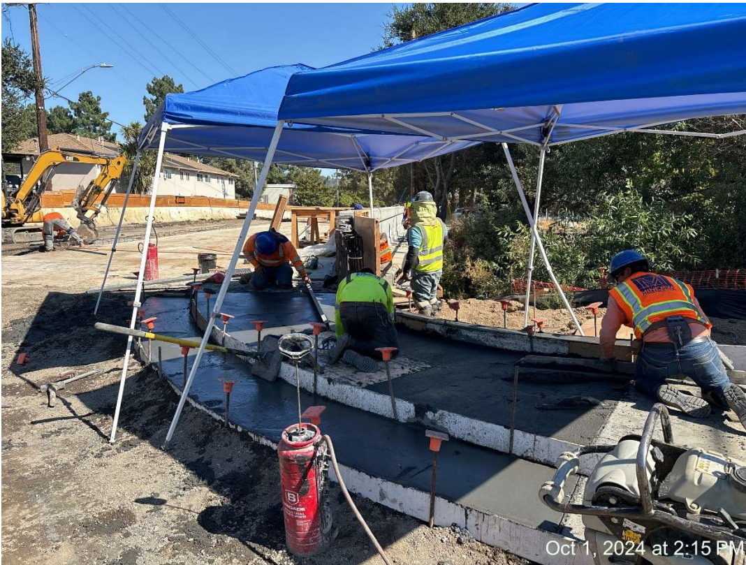
Figure 17 – Pouring Southwest Ramp (Type C)
