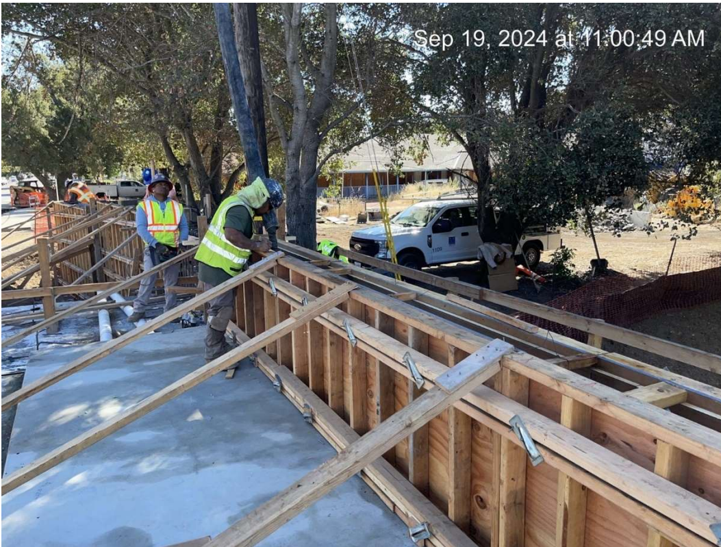
Figure 13 – Pouring Bridge Barrier.
