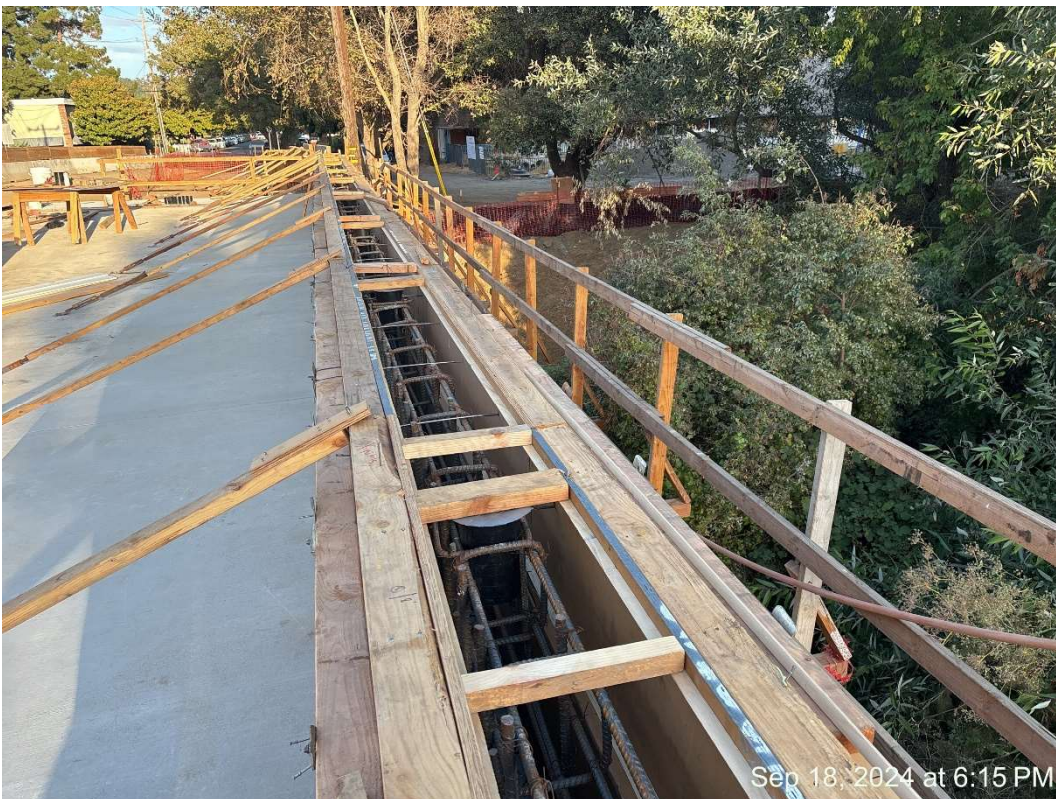
Figure 12 – Ready for Type 732 SW Barrier Pour.
