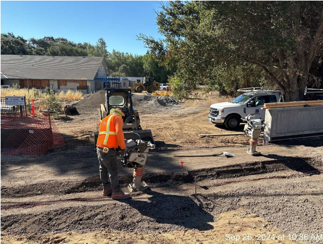
Figure 9 – Compacting base for the Sidewalk.
