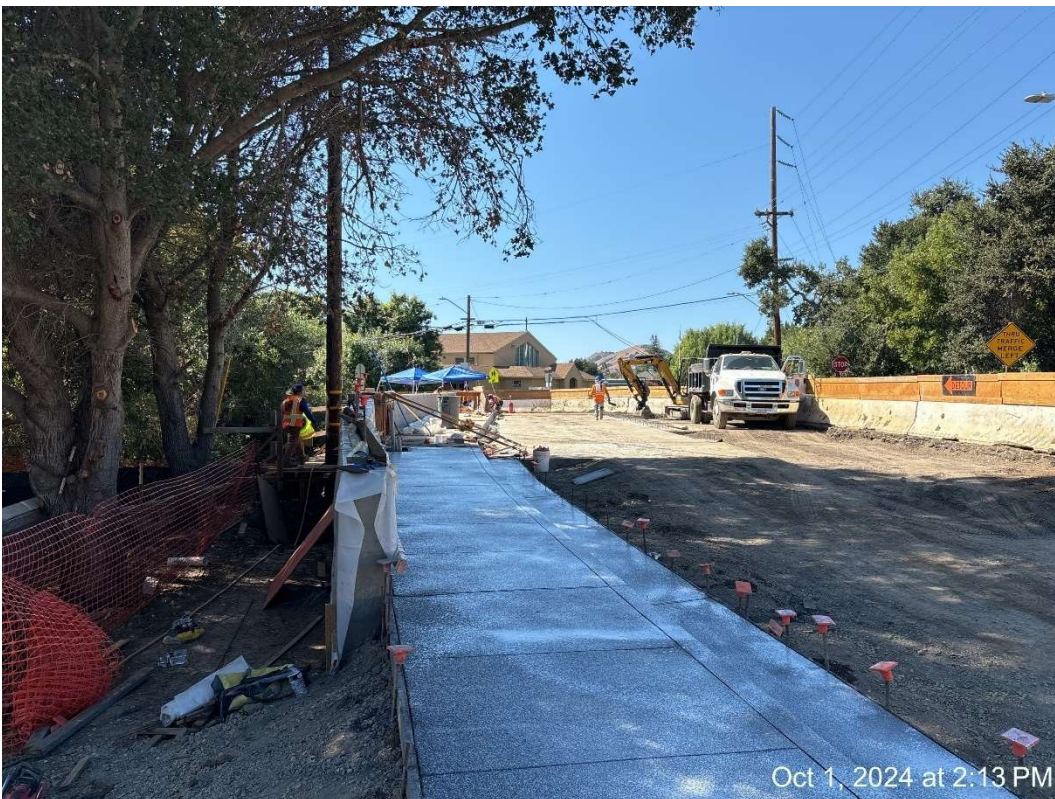
Figure 16 – Sidewalk section by Retaining Wall Poured.
