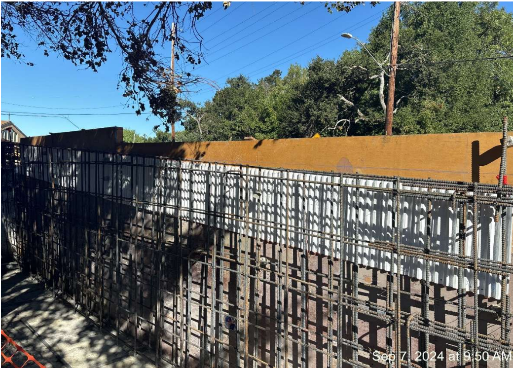
Figure 1 – Retaining Wall Stem Reinforcement complete.
