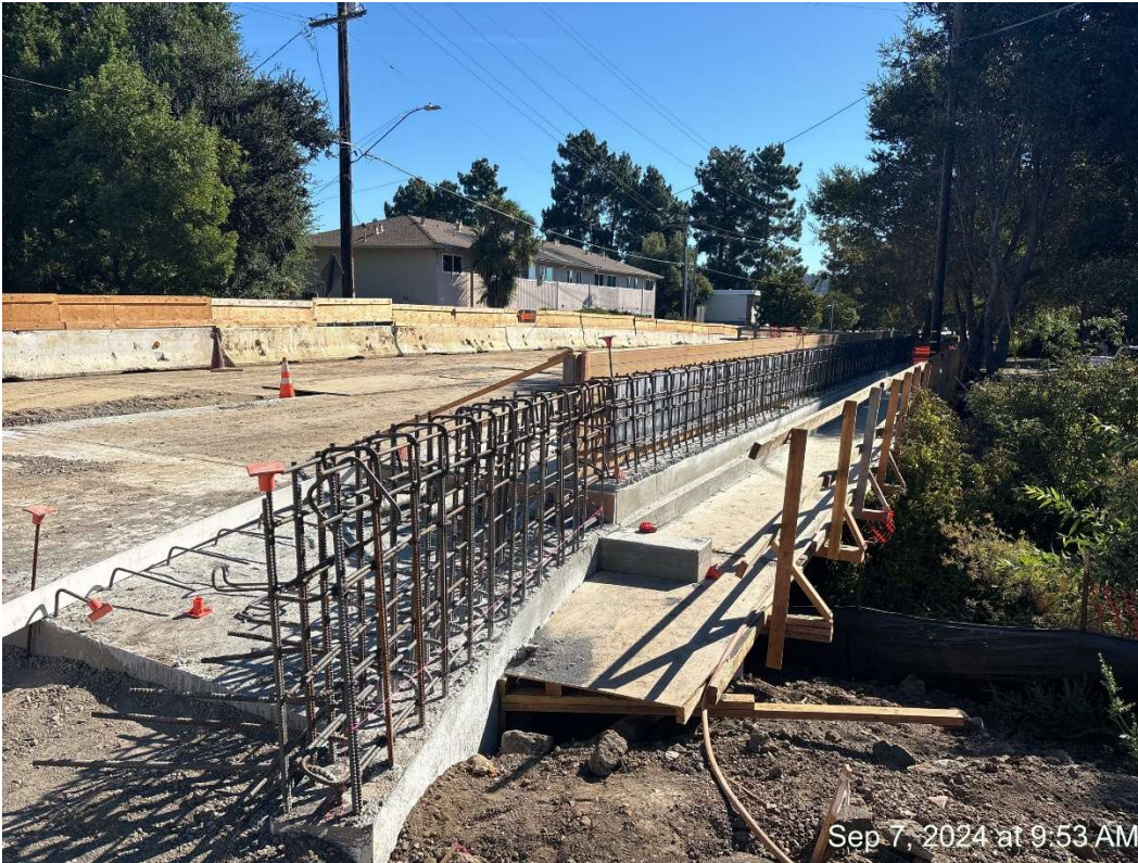
Figure 3 – Bridge Barrier Rebar almost complete.
