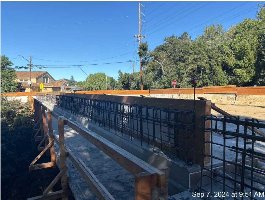
Figure 2 – Begin forming Type 732 Bridge Barrier
