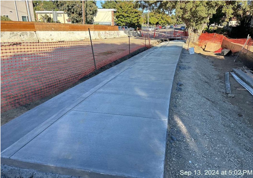
Figure 7 – Pour curb, gutter & sidewalk near Cork Oak.
