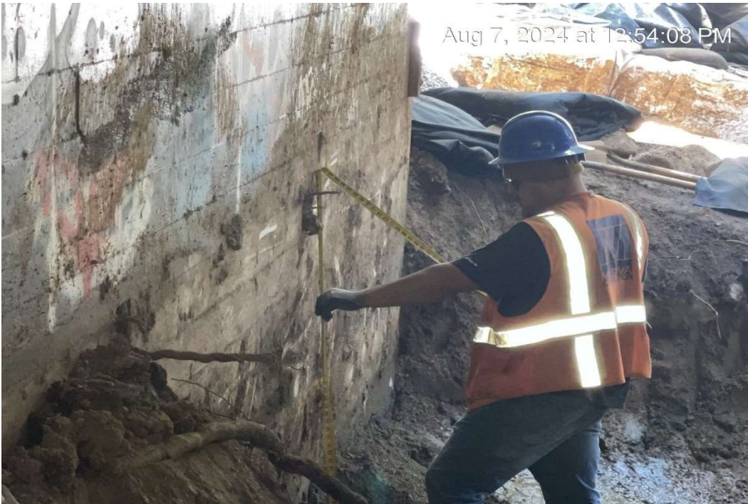
Figure 3 – Contractor measuring distance to weepholes.
