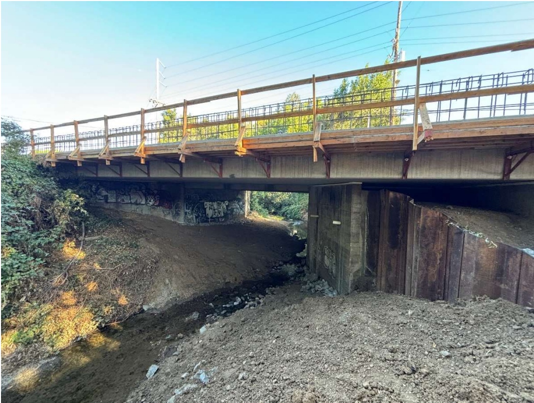
Figure 10 – Creek Restoration complete.
