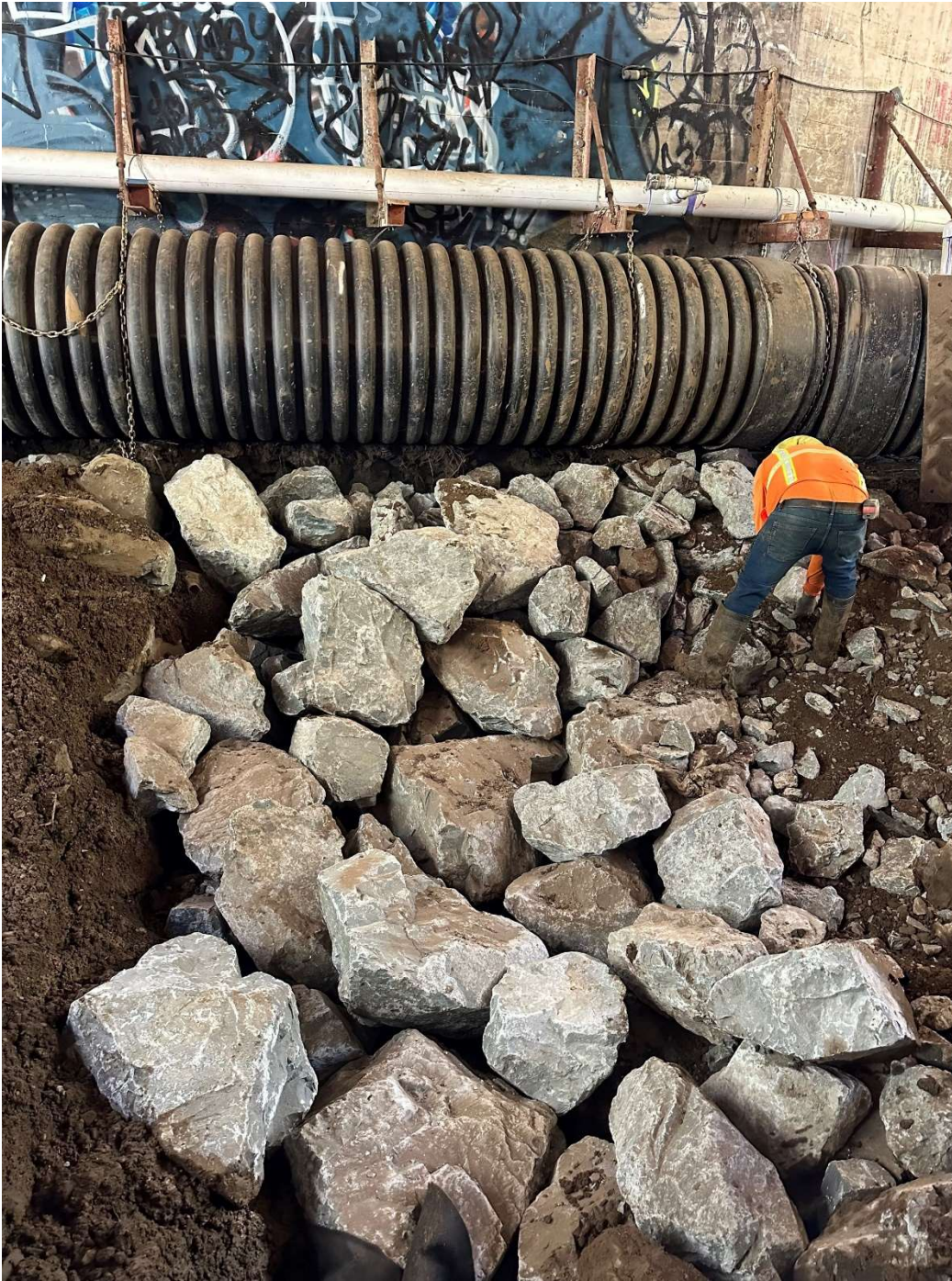
Figure 5 – Placing ¼ Ton RSP under suspended conveyance pipe.
