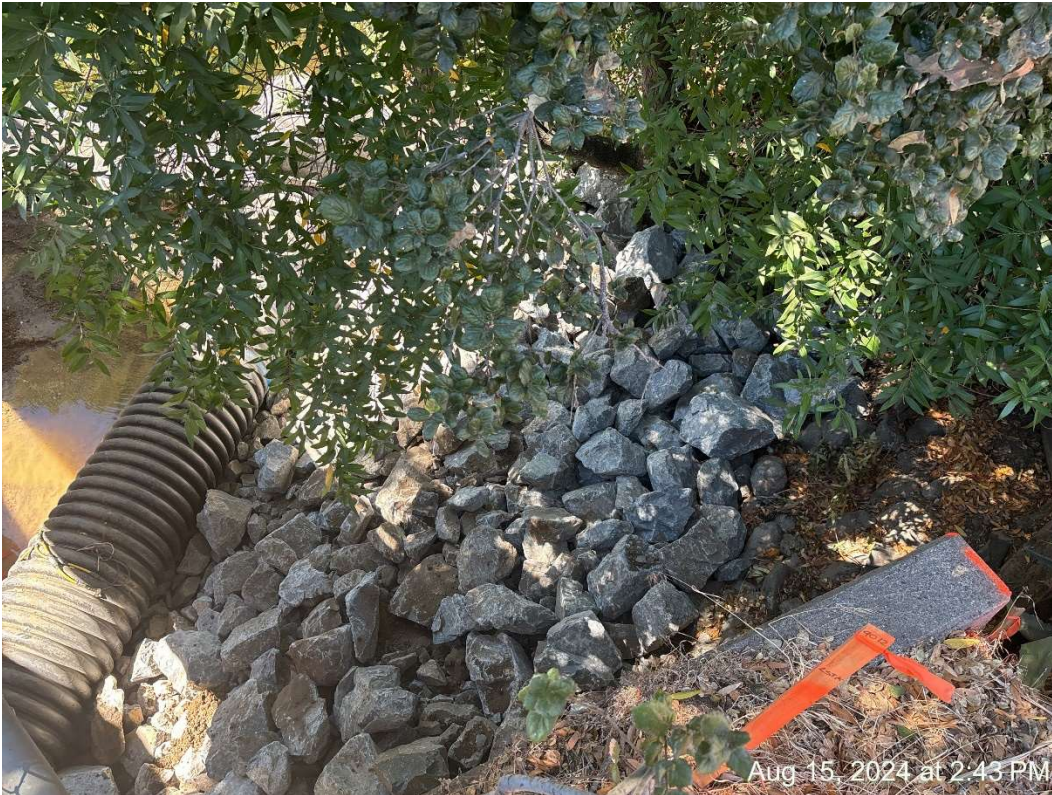
Figure 6 – RSP placed in maintenance easement.
