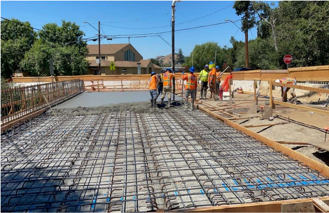
Figure 12 – Pouring Deck.
