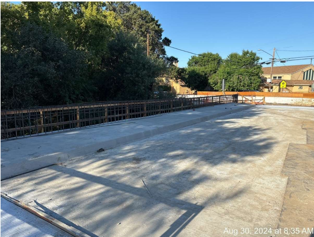
Figure 19 – Completed Approach Slabs.
