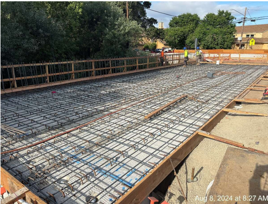
Figure 11 – Deck Reinforcement Placed.
