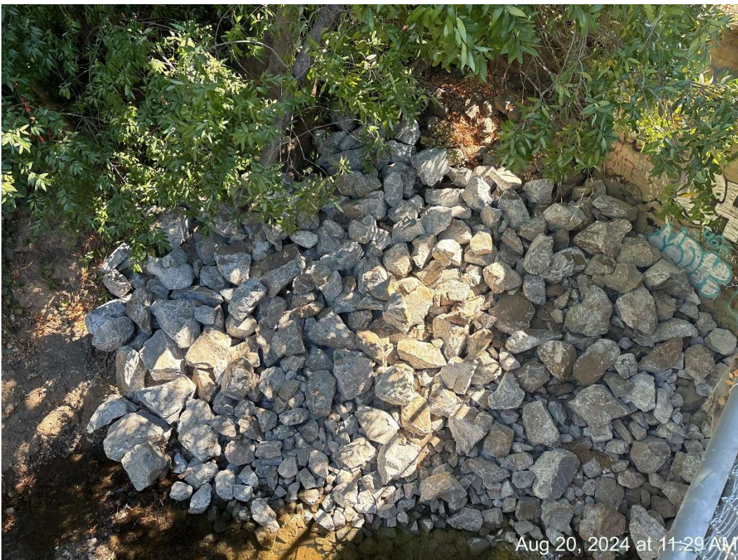
Figure 7 – RSP placed in maintenance easement.
