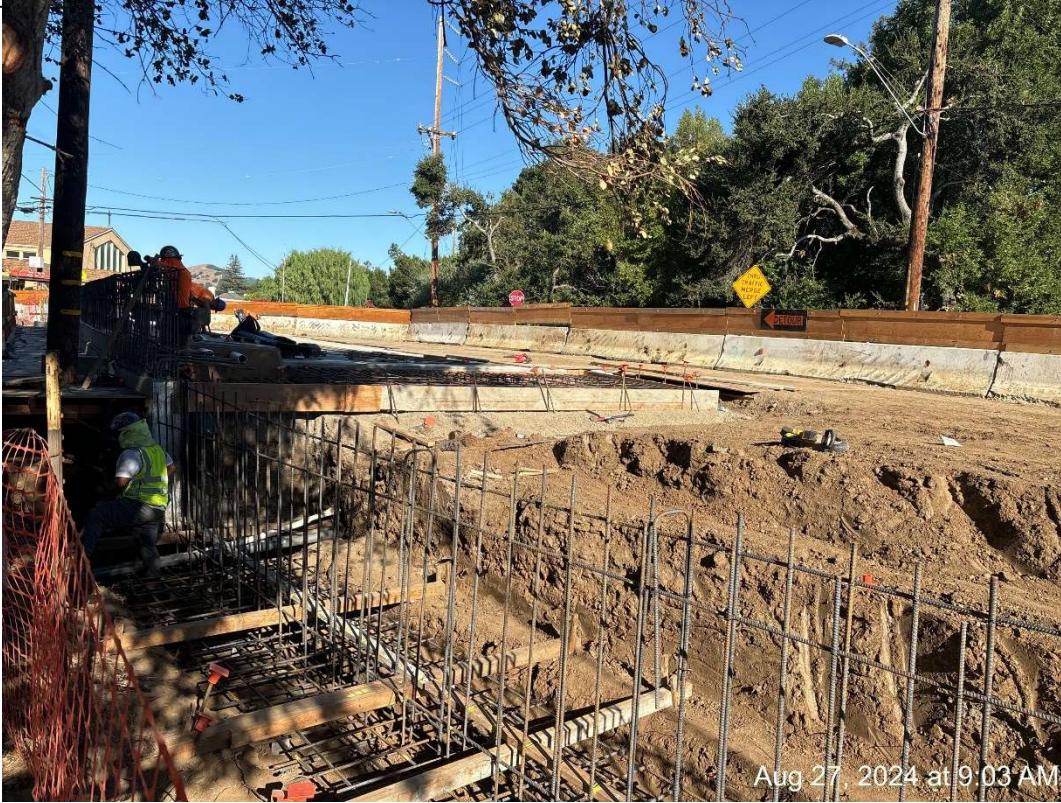
Figure 20 – Retaining Wall Reinforcement complete in footing.
