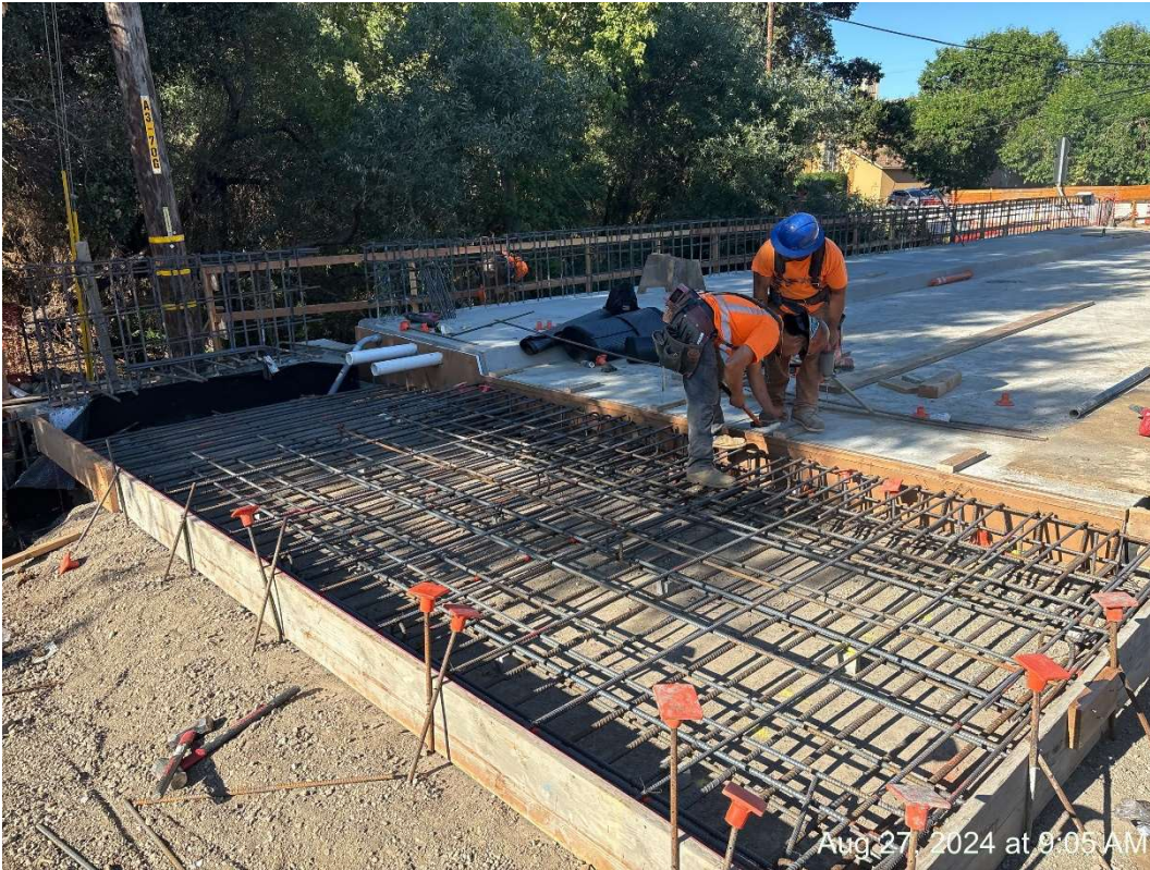
Figure 18 – Bar Reinforcement for Approach Slabs.
