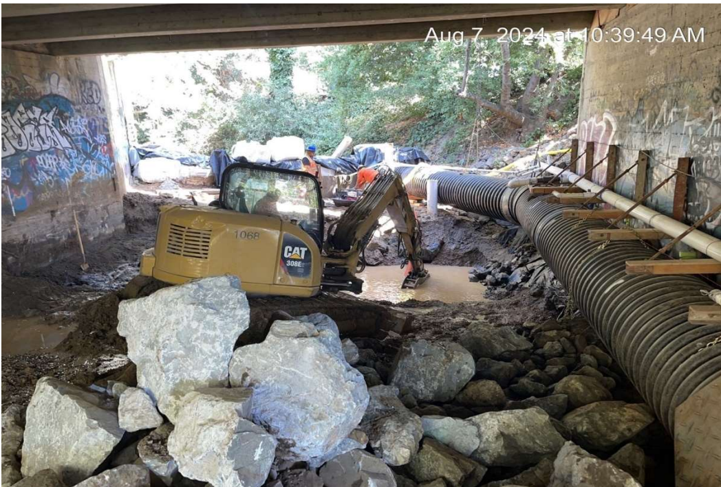
Figure 2 – Contractor excavating and dewatering to place ¼ Ton RSP.
