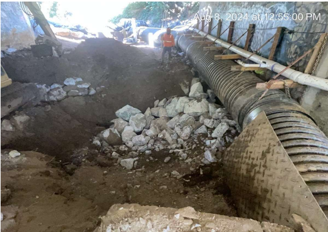
Figure 4 – Placing ¼ Ton RSP.
