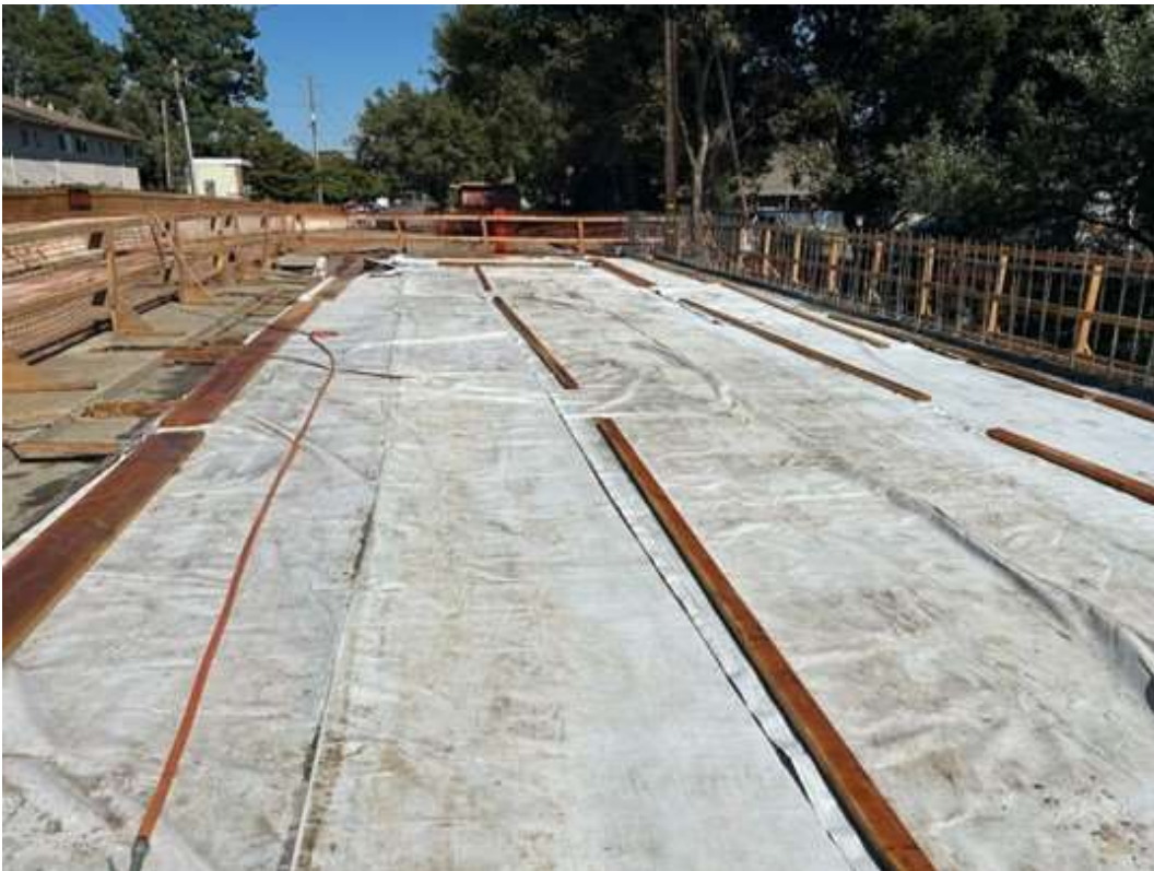
Figure 13 – Curing Deck – Water Cure.
