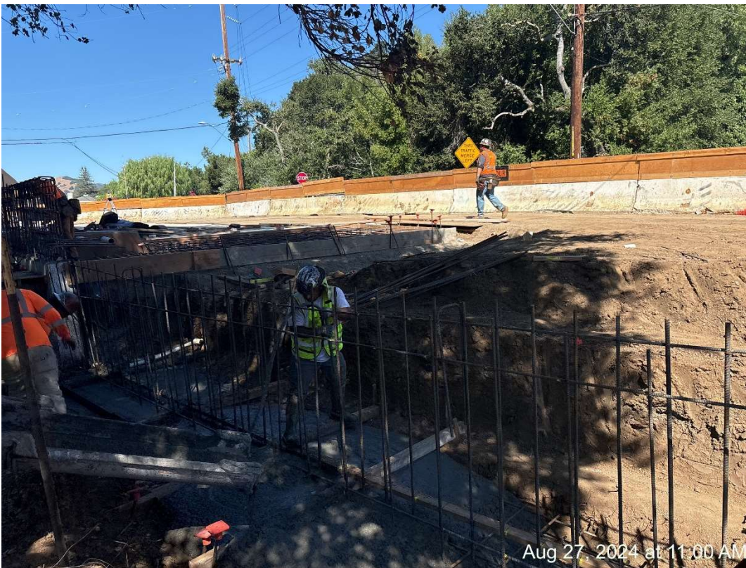
Figure 21 – Pour Retaining Wall Footing.
