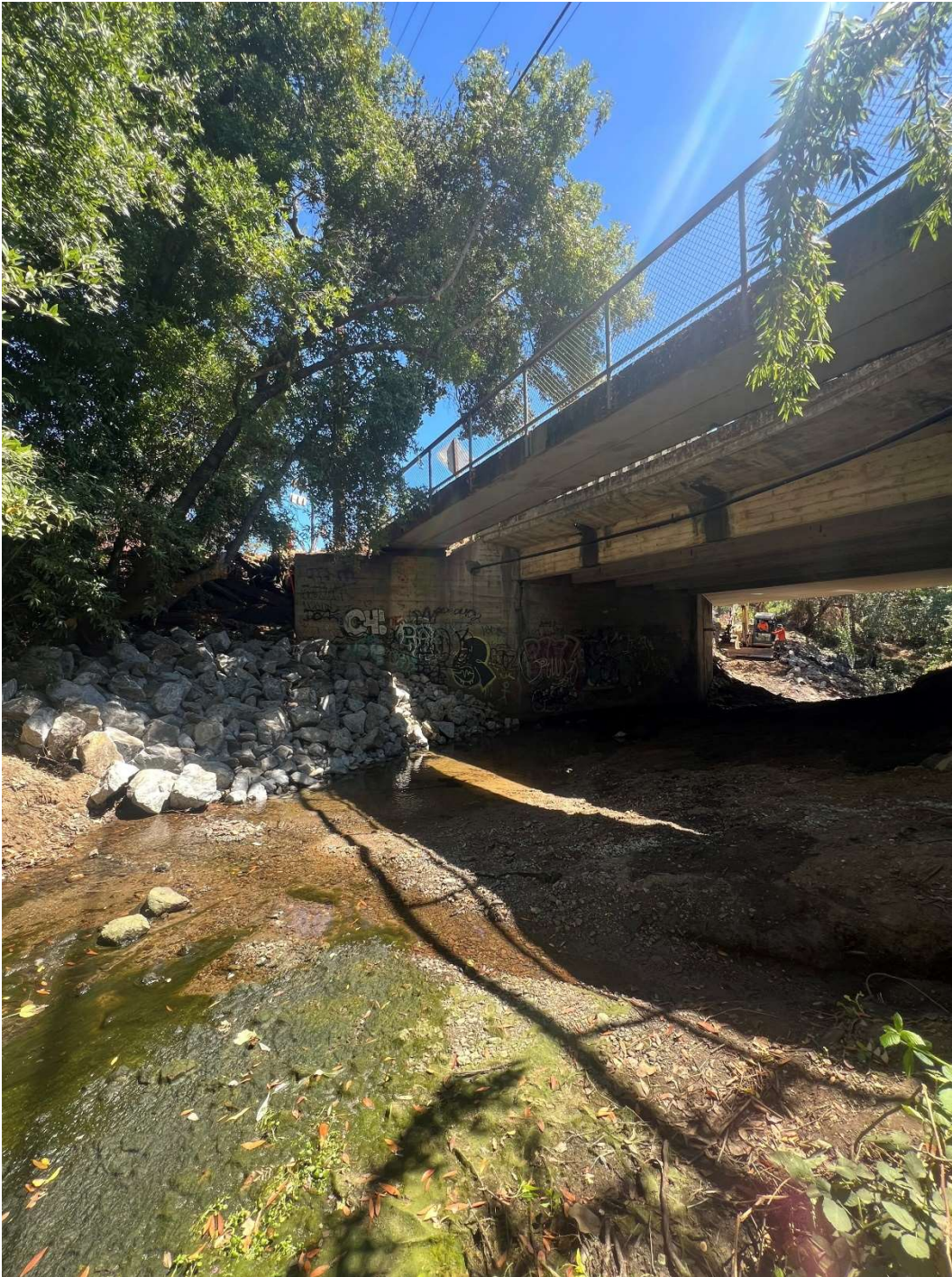
Figure 8 – Cofferdam removed and Creek Restoration.
