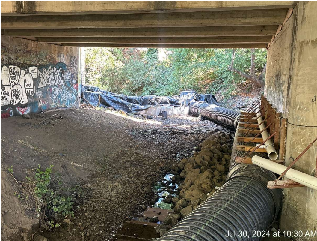
Figure 19 – Upstream cofferdam complete.
