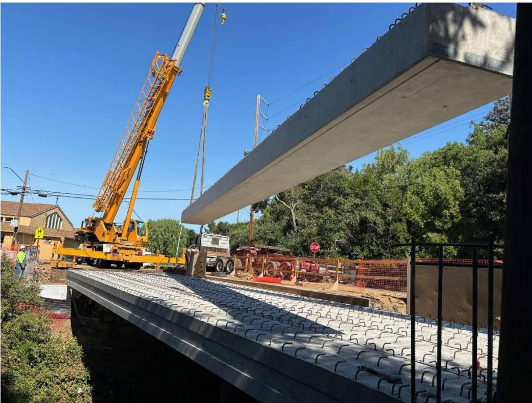
Figure 10 – Flying in last Deck Unit.
