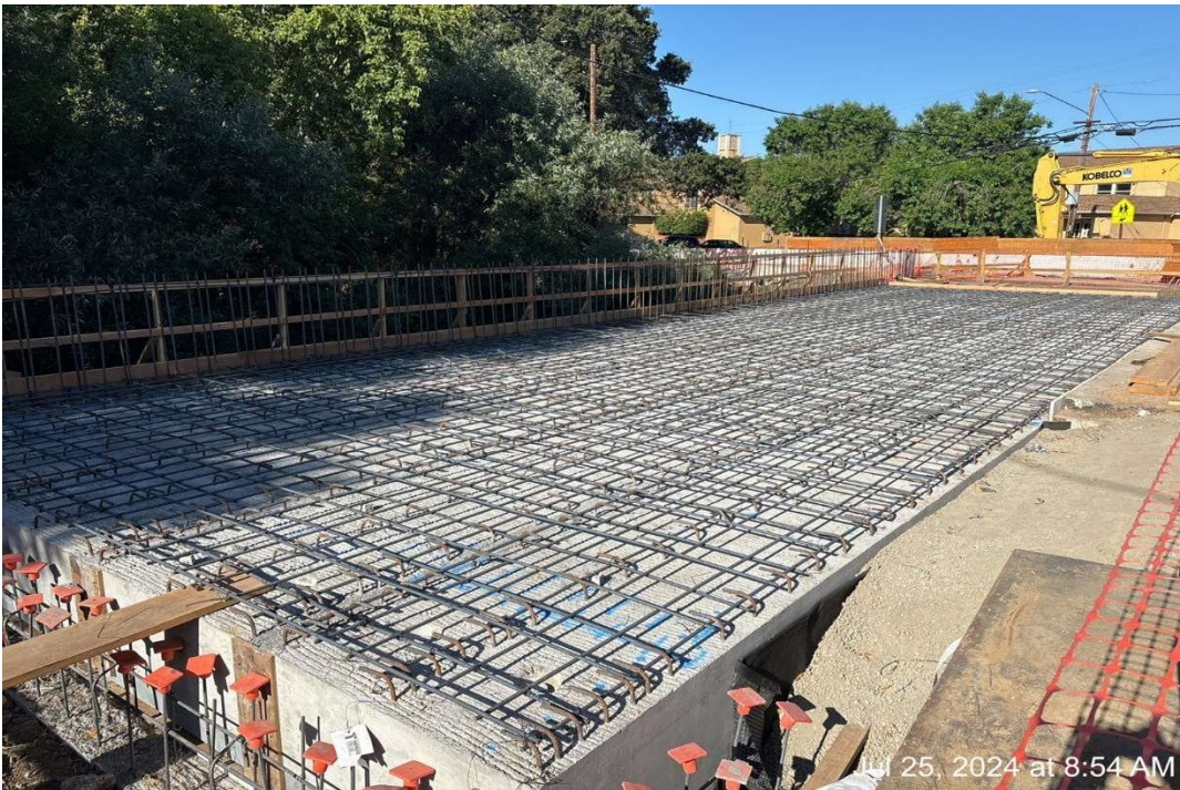
Figure 15 – Deck Bar Reinforcement Placement complete.
