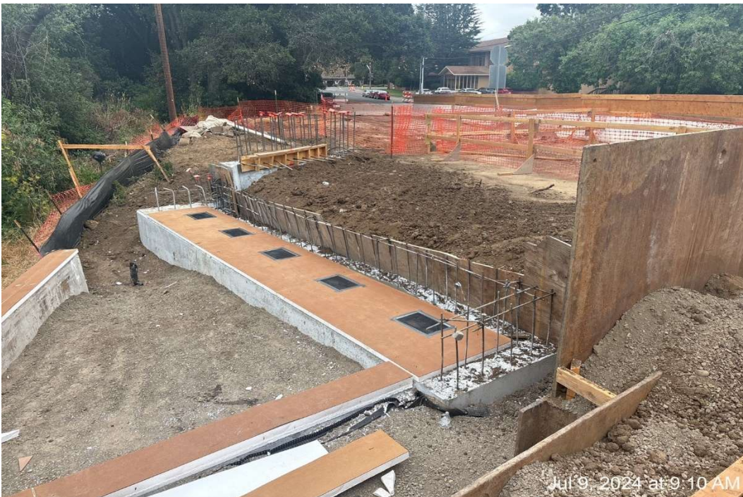
Figure 2 – Installing Bearing Pads Abutment 1.
