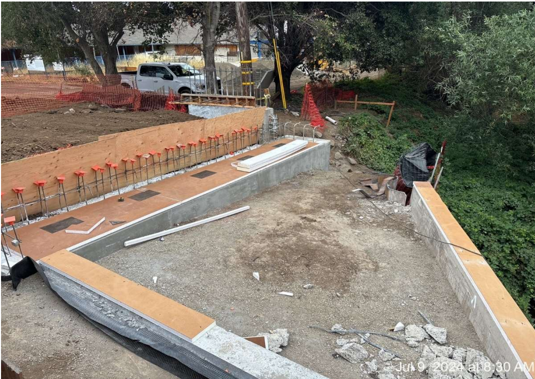
Figure 1 – Installing Bearing Pads Abutment 2.
