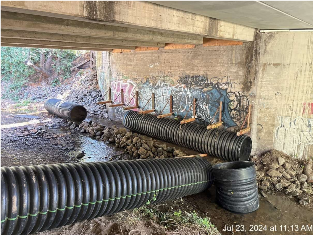
Figure 17 – Begin Creek Diversion.
