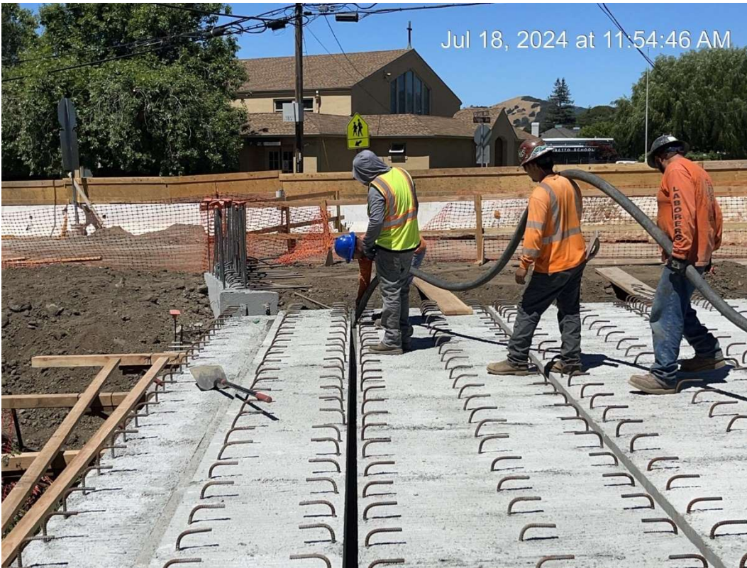
Figure 13 – Pouring Grout into Keyways between Slab Units.
