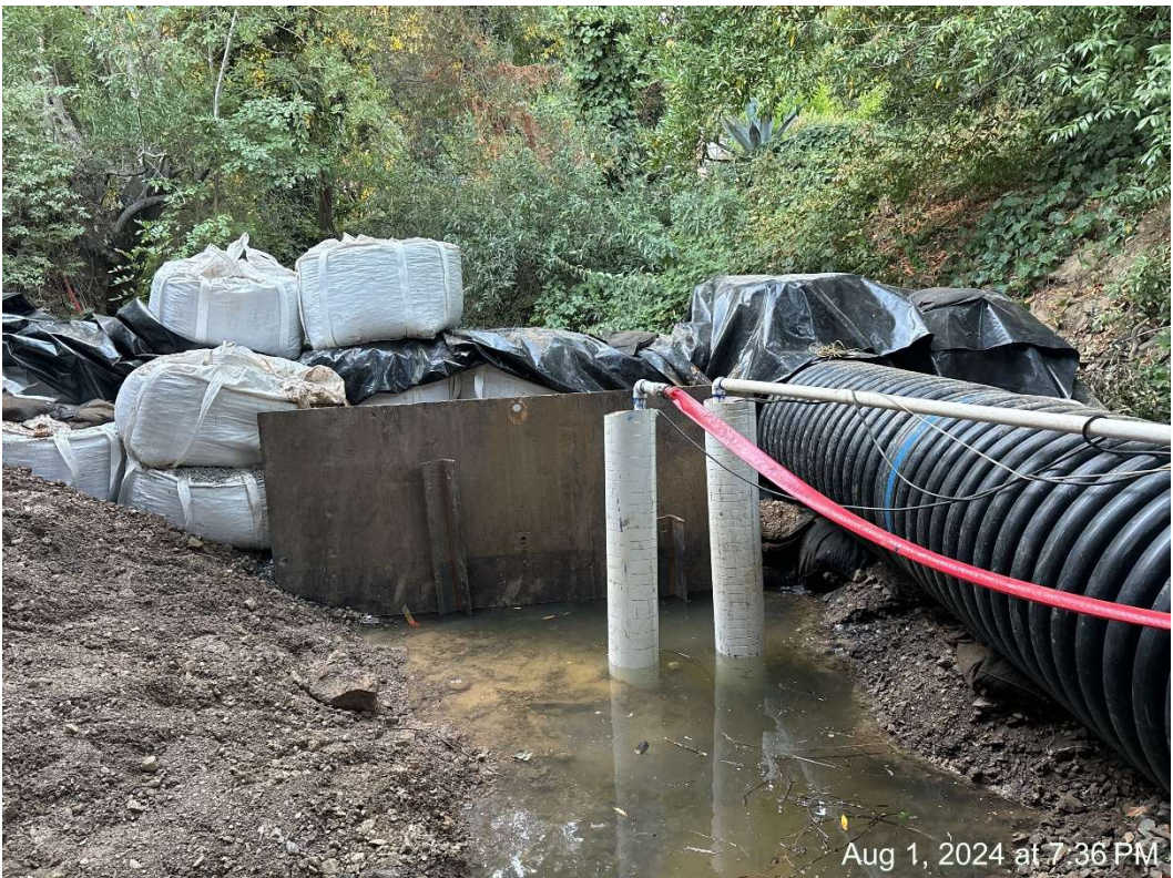
Figure 20 – Begin dewatering between cofferdams.
