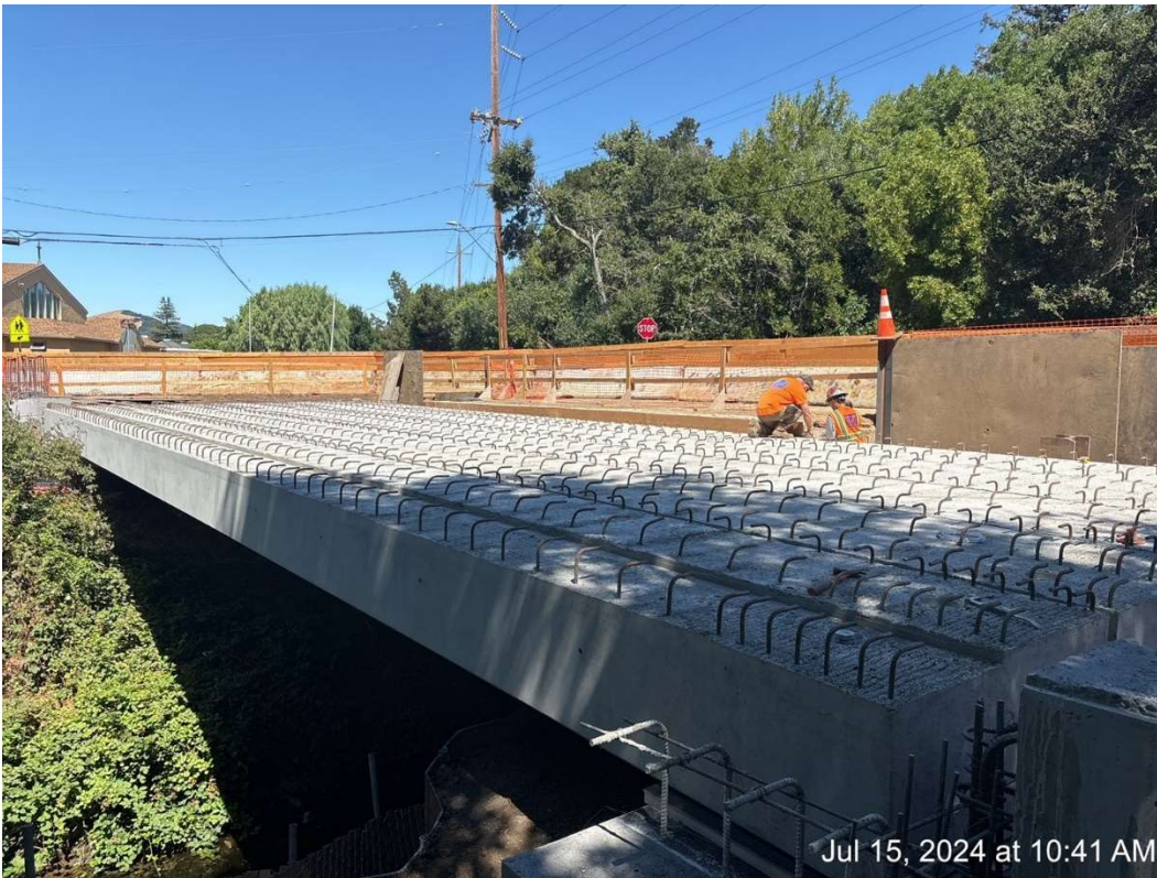
Figure 11 – Girder Placement complete.
