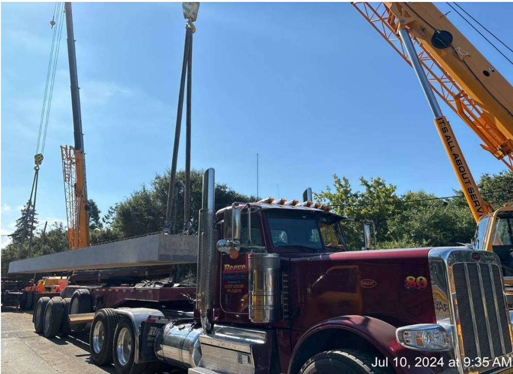
Figure 5 – Precast Voided Deck Slab Unit being hoisted by Bragg Crane
