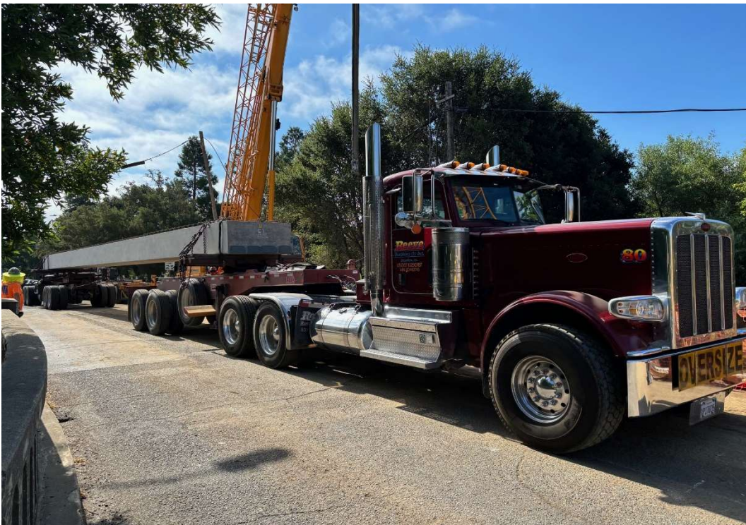
Figure 4 – Reese Trucking delivering Precast Voided Deck Slab Unit from Confab LLC.
