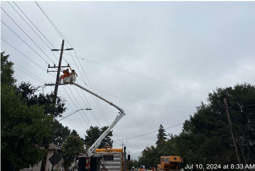
Figure 3 – The West Coast’s greatest Utility Company PG&E removing Guy Wire.
