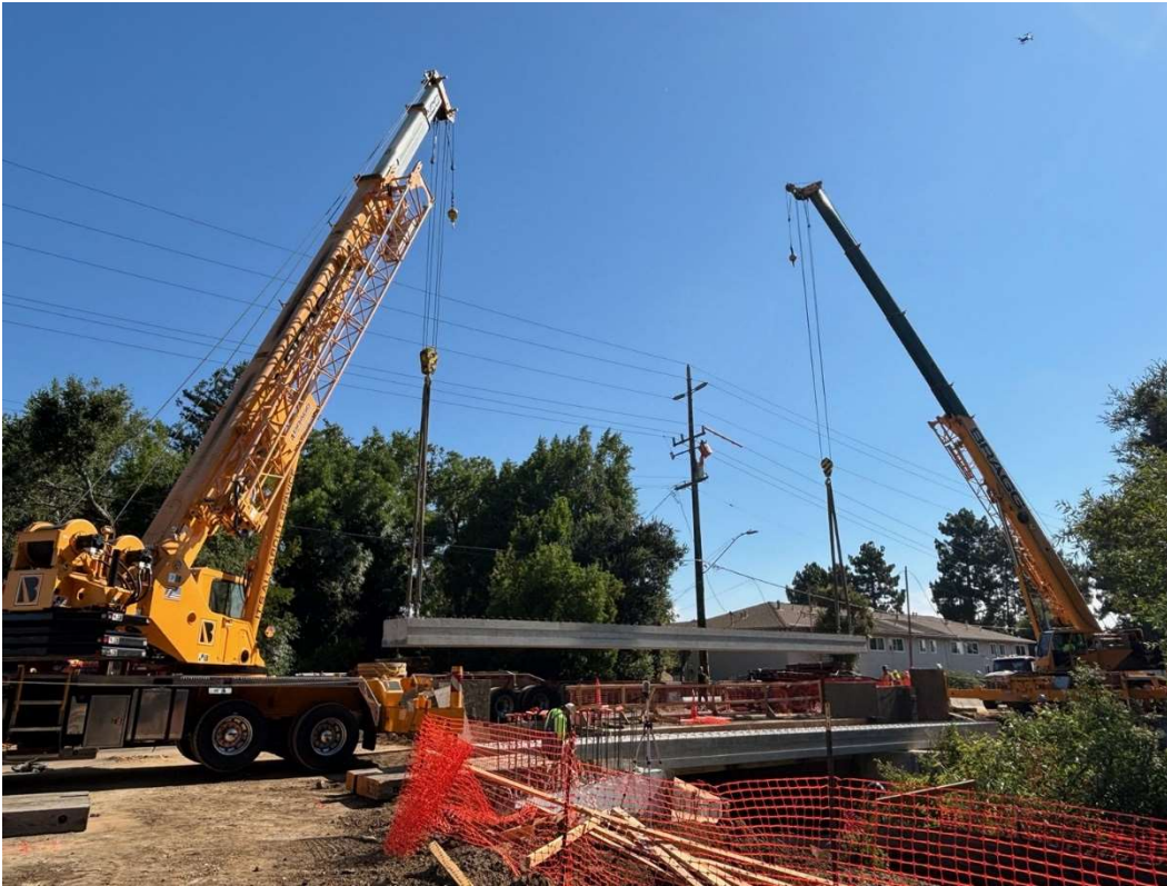
Figure 7 – Precast Voided Deck Slab Unit being erecting 2 nd girder into place.
