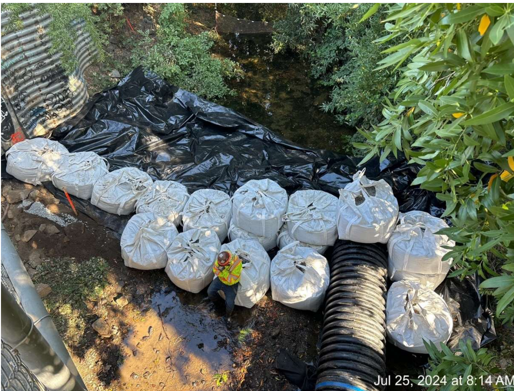
Figure 18 – Installing Upstream Cofferdam.
