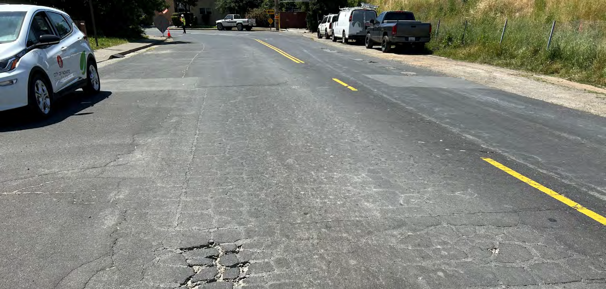
Armstrong Ave, PCI = 24 Treatment: Surface Reconstruction
