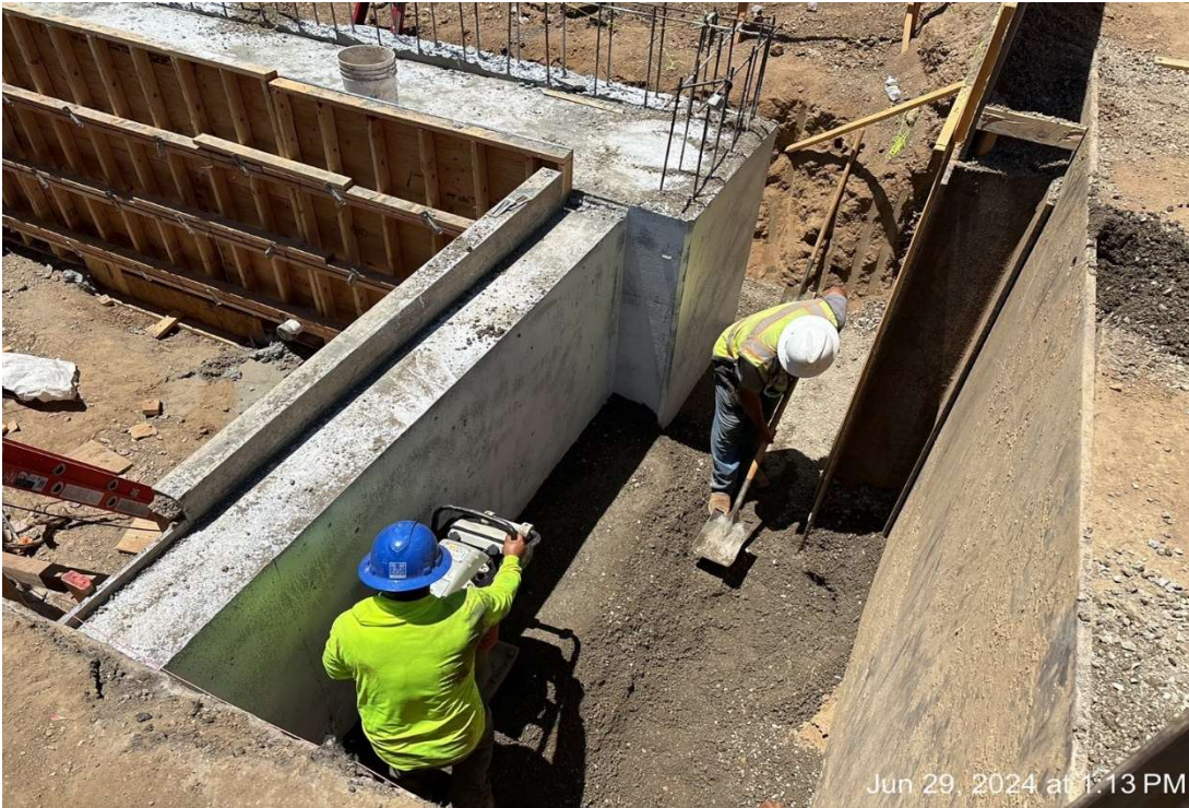
Figure 21 – Backfilling at Abutment 2.
