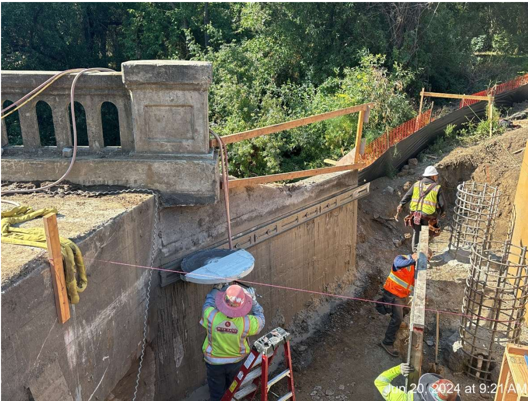
Figure 6 – Sawcutting wingwall near Abutment 2.
