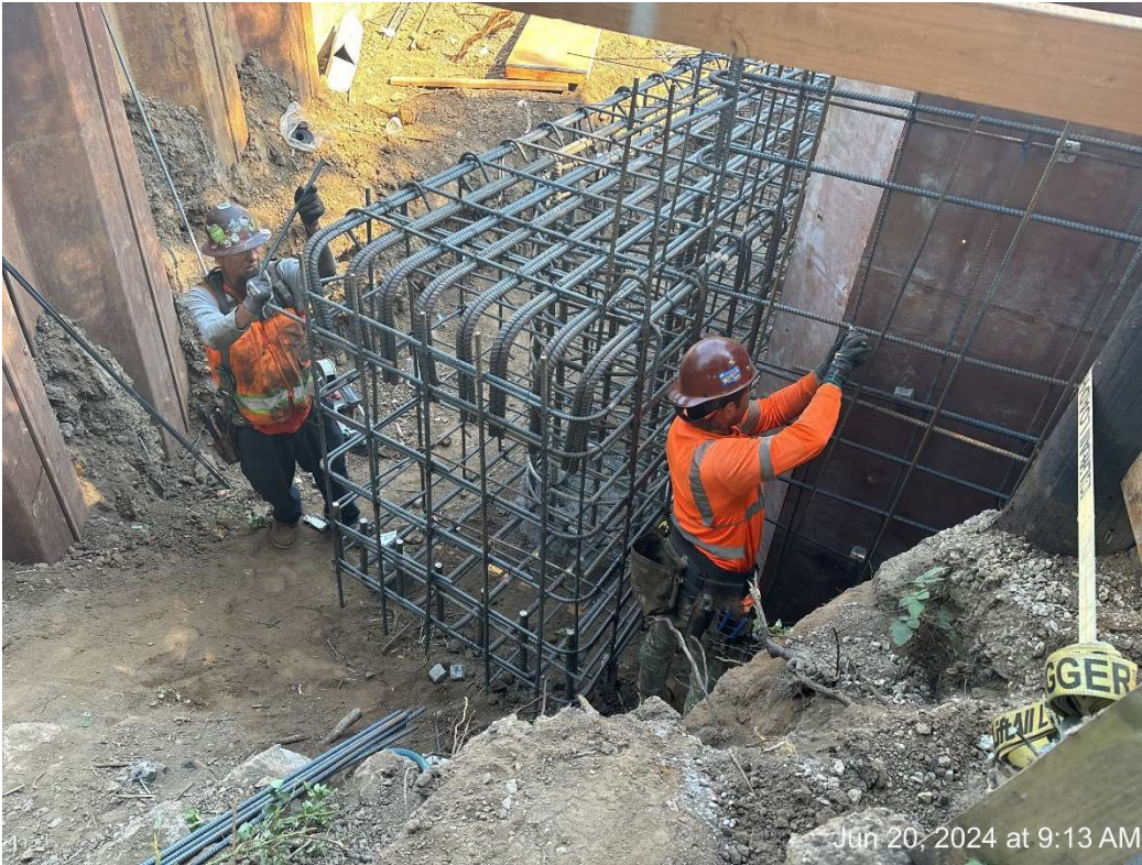
Figure 7 – Abutment 2 Bar Reinforcement Placement.
