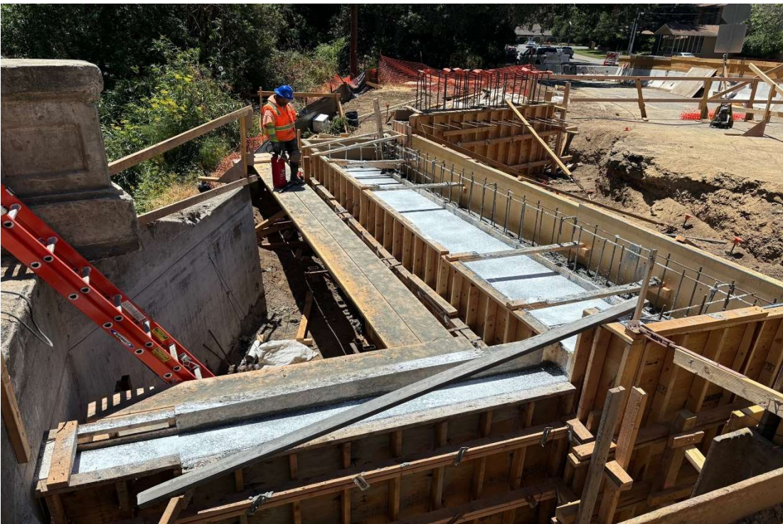
Figure 18 – Abutment 2 – Concrete Poured Out and Cure Applied.
