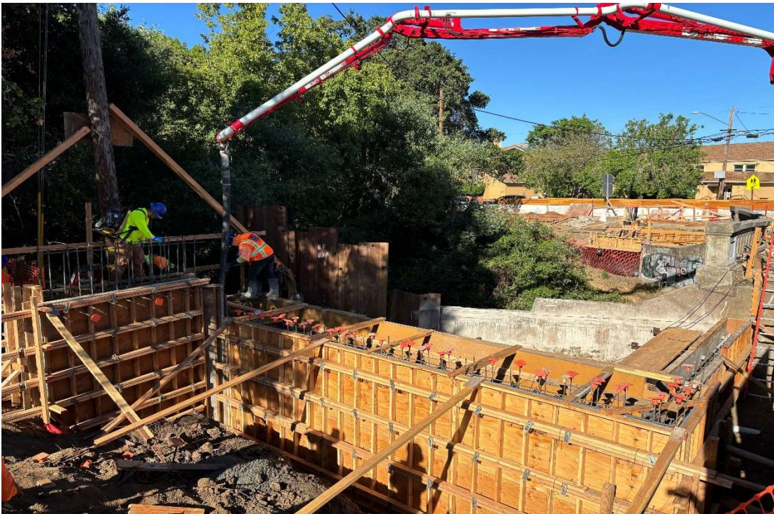
Figure 16 – Pouring Concrete at Abutment 1.
