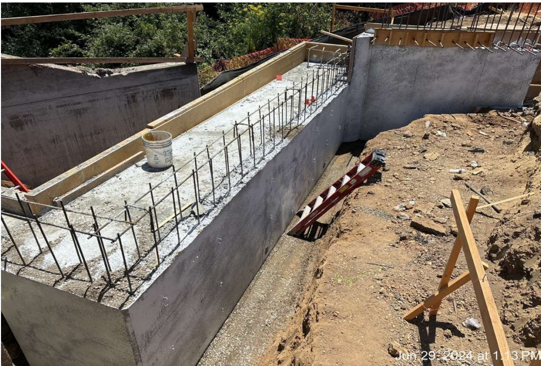
Figure 20 – Forms stripped and backfill 2ft – Abutment 2.
