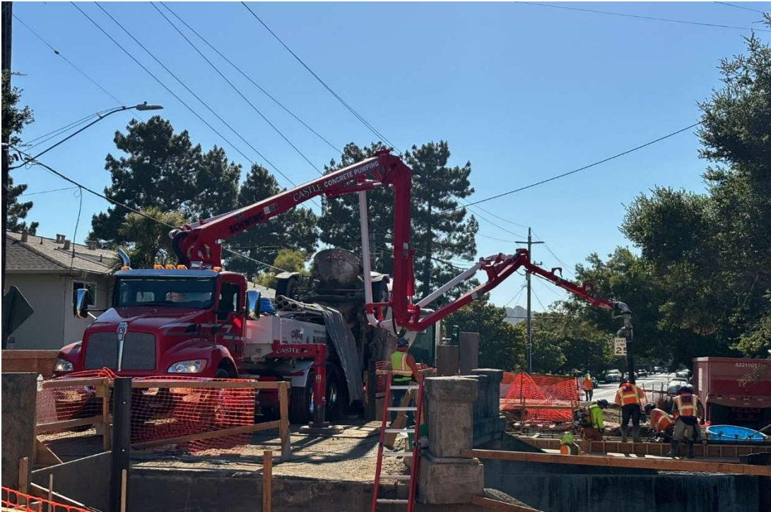
Figure 15 – Pouring Concrete at Abutment 1.
