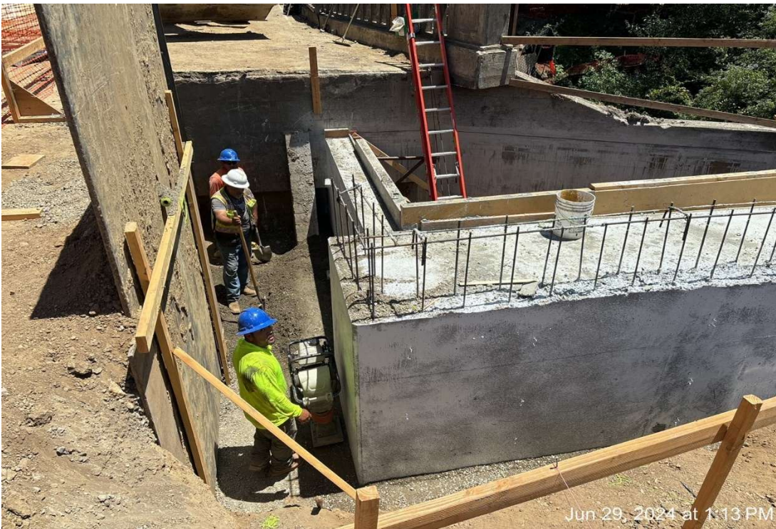
Figure 22 – Backfilling at Abutment 2.
