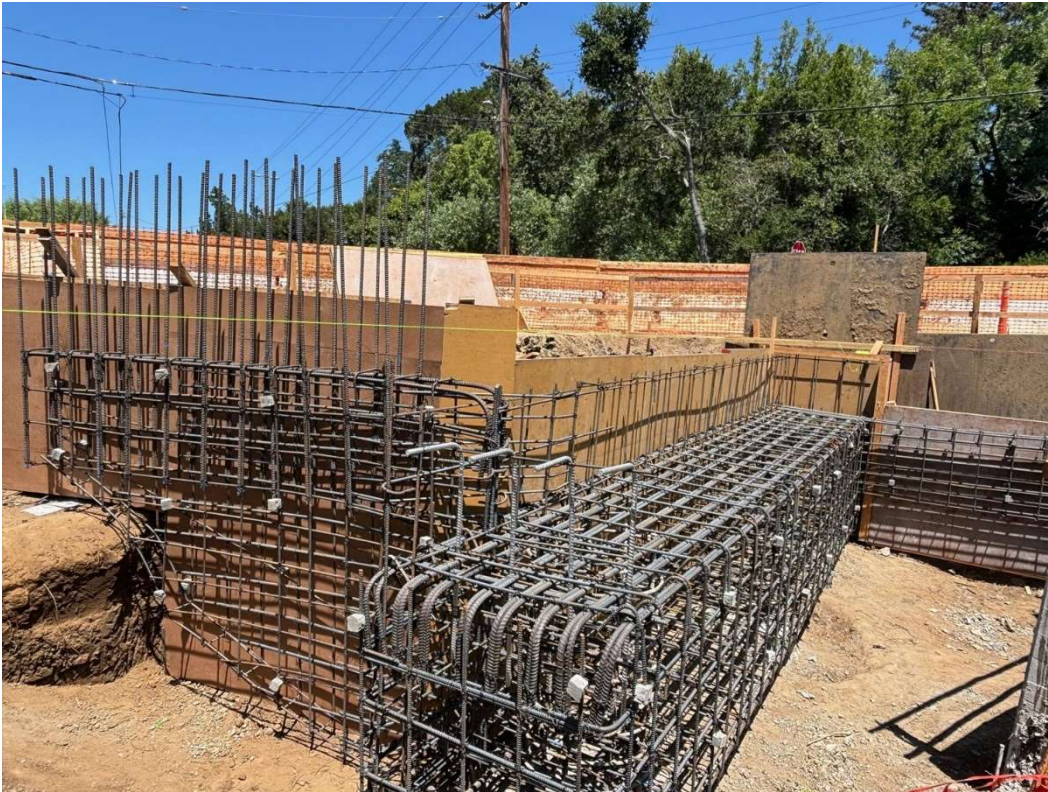
Figure 13 – Bar Reinforcement Placed at Abutment 1.
