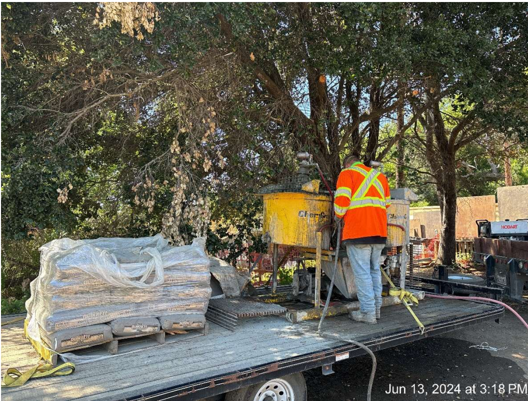
Figure 3 – Grouting Inspection Tubes.
