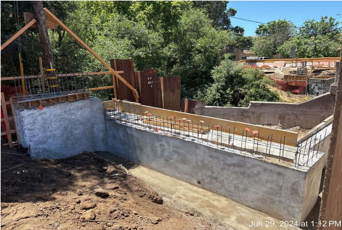
Figure 19 – Forms stripped and backfill 2ft – Abutment 2.
