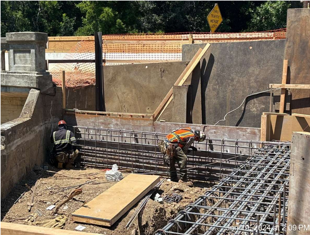
Figure 11 – Interior grade beam bar reinforcement.
