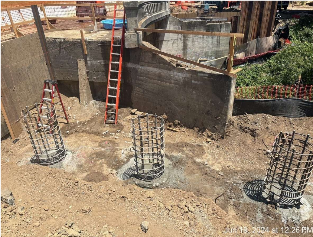
Figure 5 – Finished Grouting of Inspection Tubes at Abutment 1.
