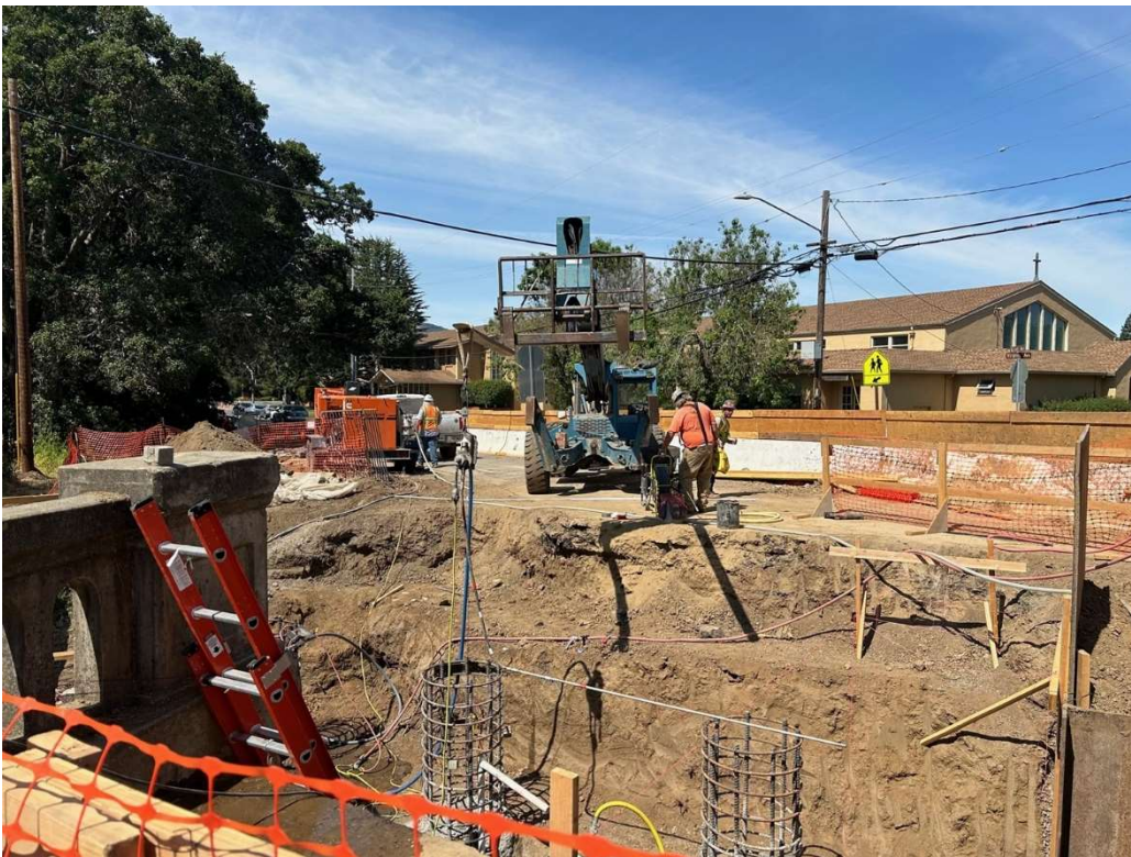
Figure 2 – American Water Jetting Repair of Abutment 1 – Pile #2.
