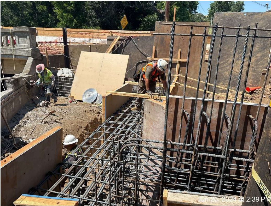
Figure 8 – Abutment 2 Bar Reinforcement Placement.
