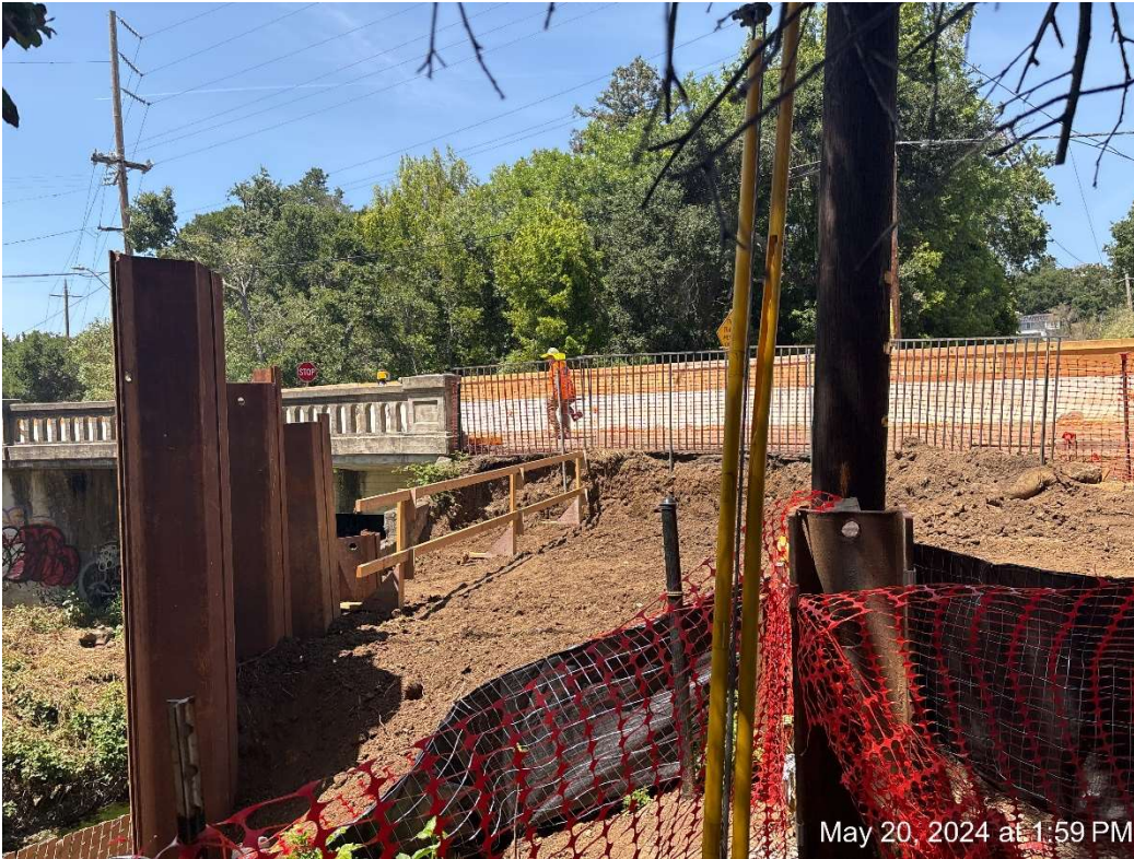
Figure 7 – Minerva installing Abutment 2 Sheetpile Shoring.
