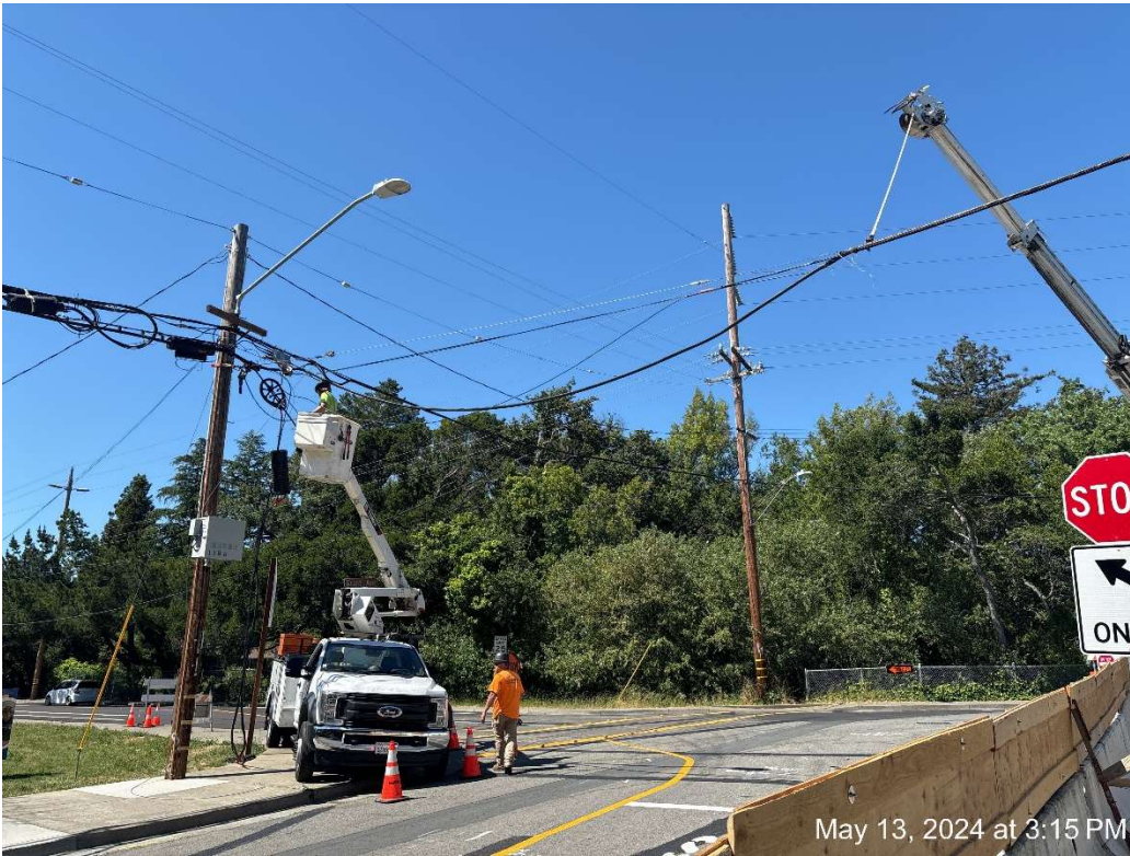
Figure 1 – Frontier Relocating OH Communication Line.
