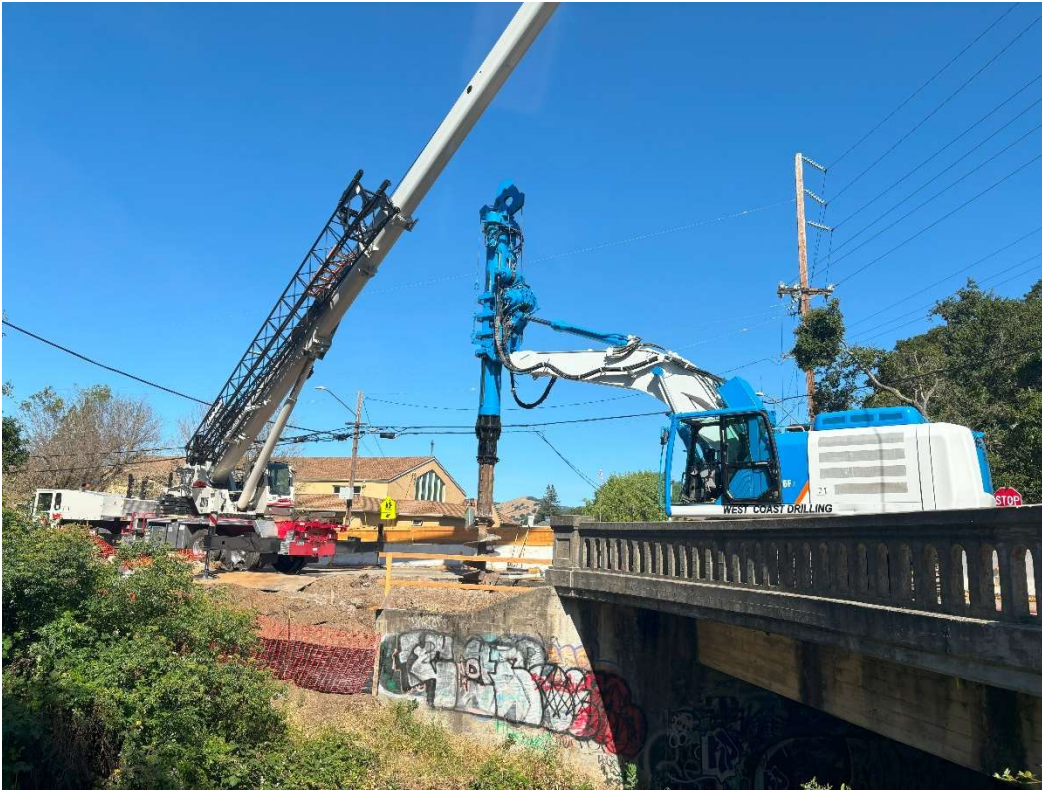
Figure 11 – West Coast Drilling Starting Drilling Operations at Abutment 1.
