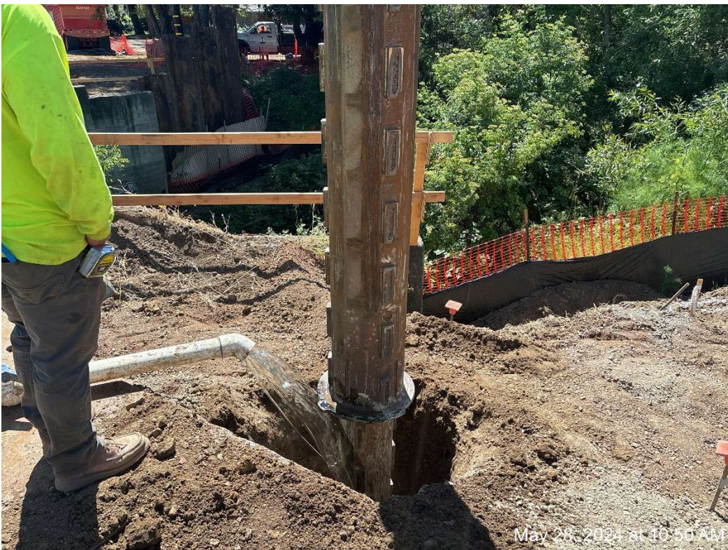
Figure 12 – West Coast Drilling adding synthetic slurry.
