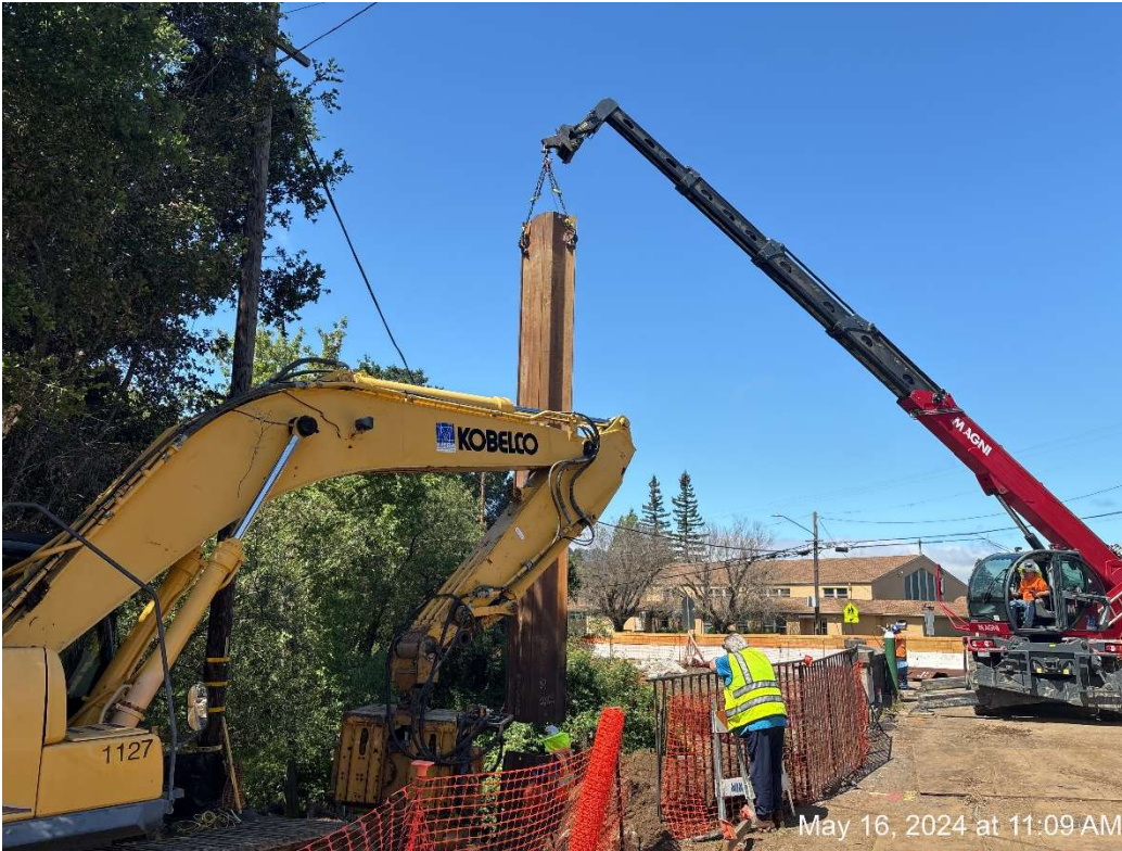
Figure 5 – Minerva installing Abutment 2 Sheetpile Shoring.
