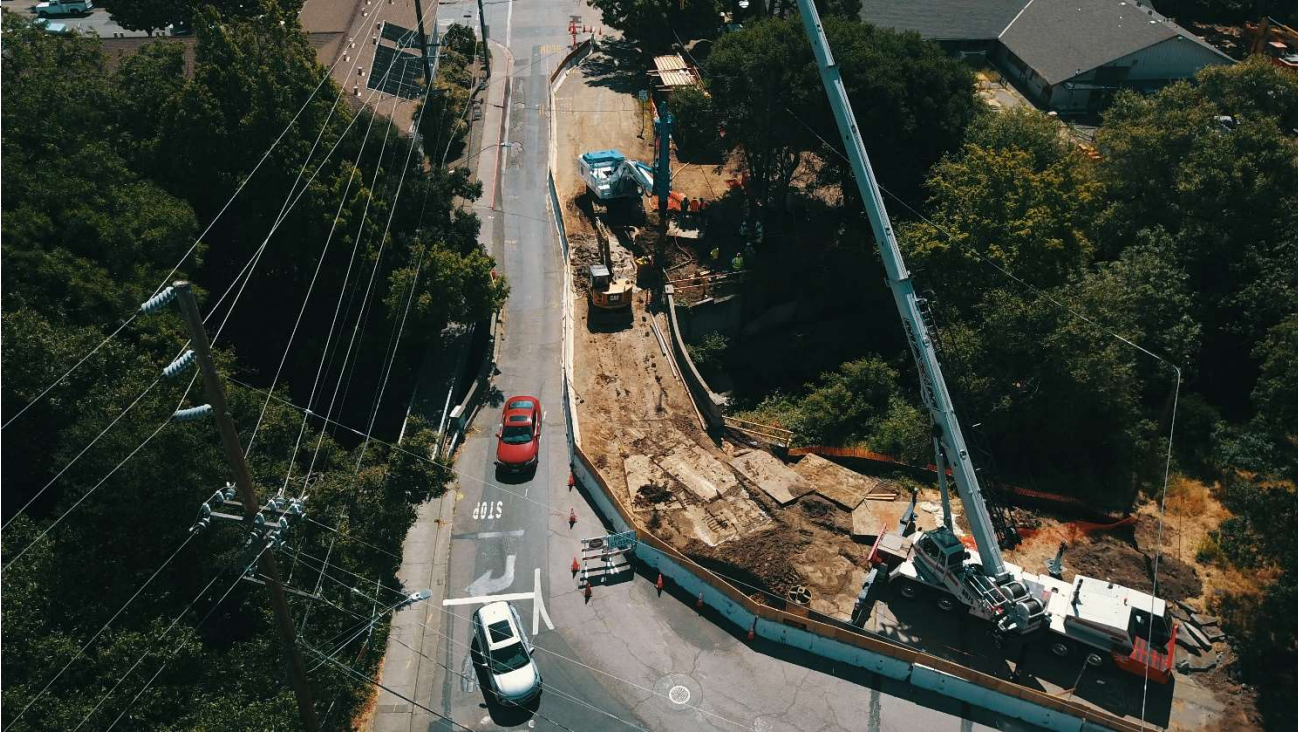
Figure 17 – Drone Picture of Drilling at Abutment 2 looking EB on Grant Ave.
