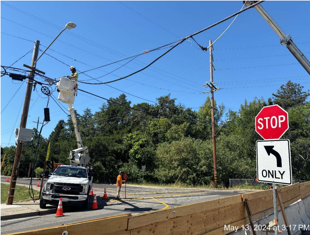
Figure 3 – Frontier Relocating OH Communication Line.
