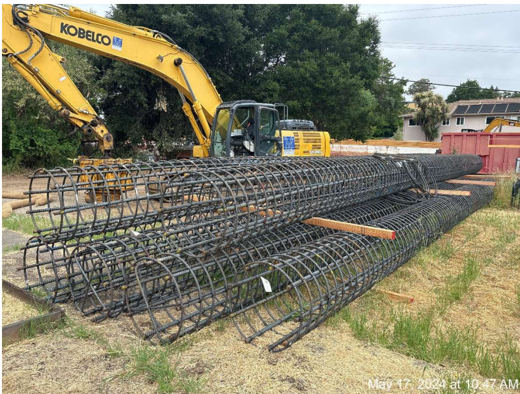
Figure 10 – CIDH Pile Rebar Cages on site.
