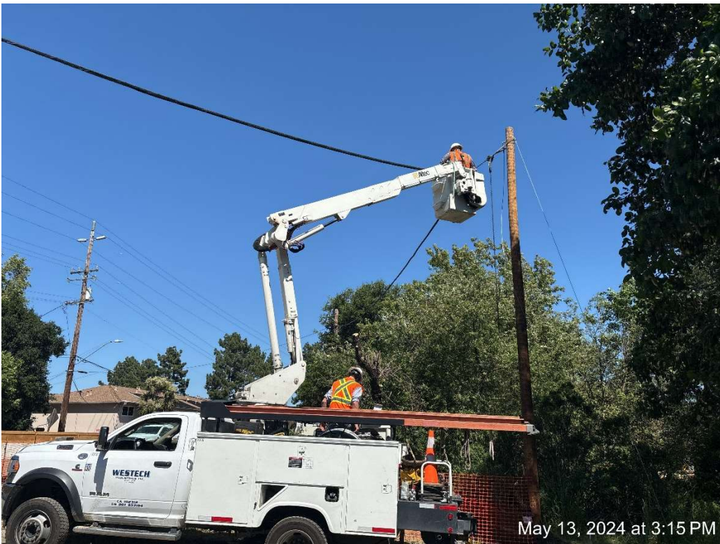
Figure 2 - Frontier Relocating OH Communication Line.
