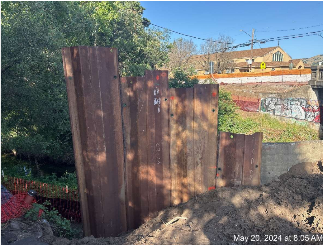
Figure 8 – Minerva installing Abutment 2 Sheetpile Shoring.
