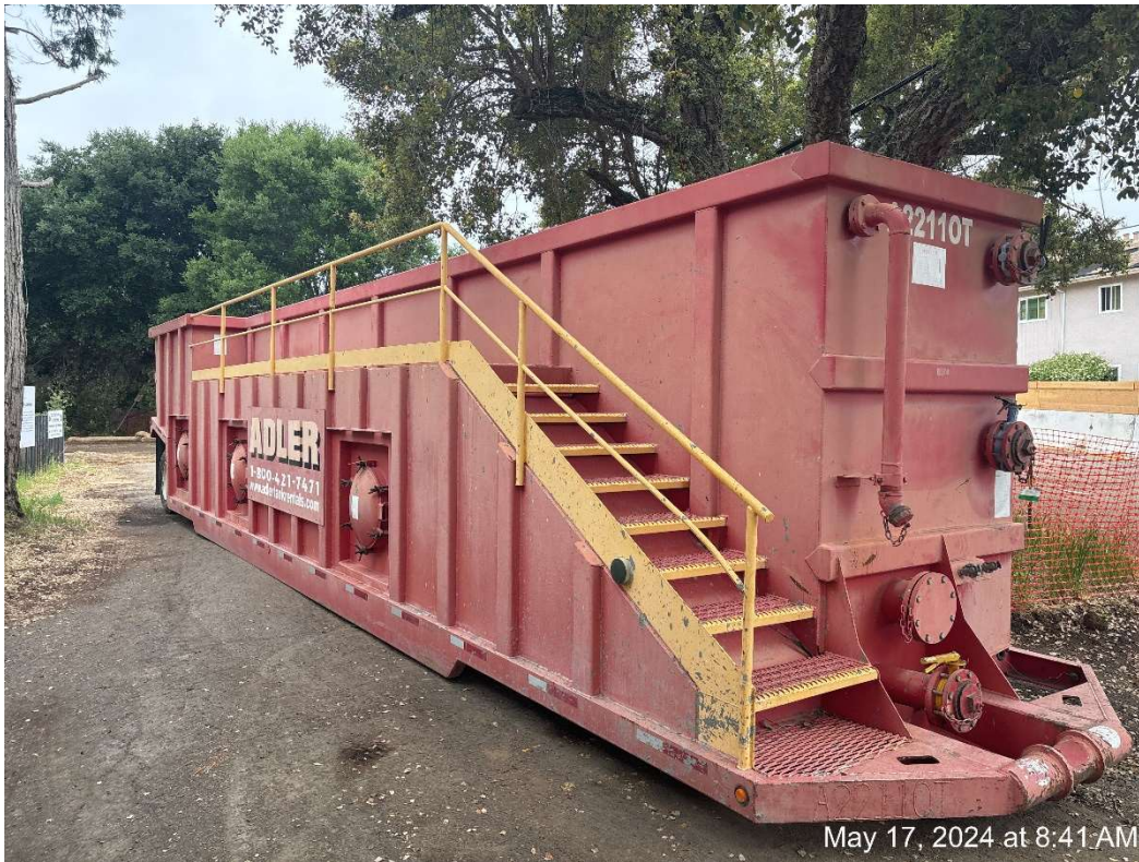
Figure 9 – West Coast Drilling Mobilizing in (20,000 Gallon Baker Tank).
