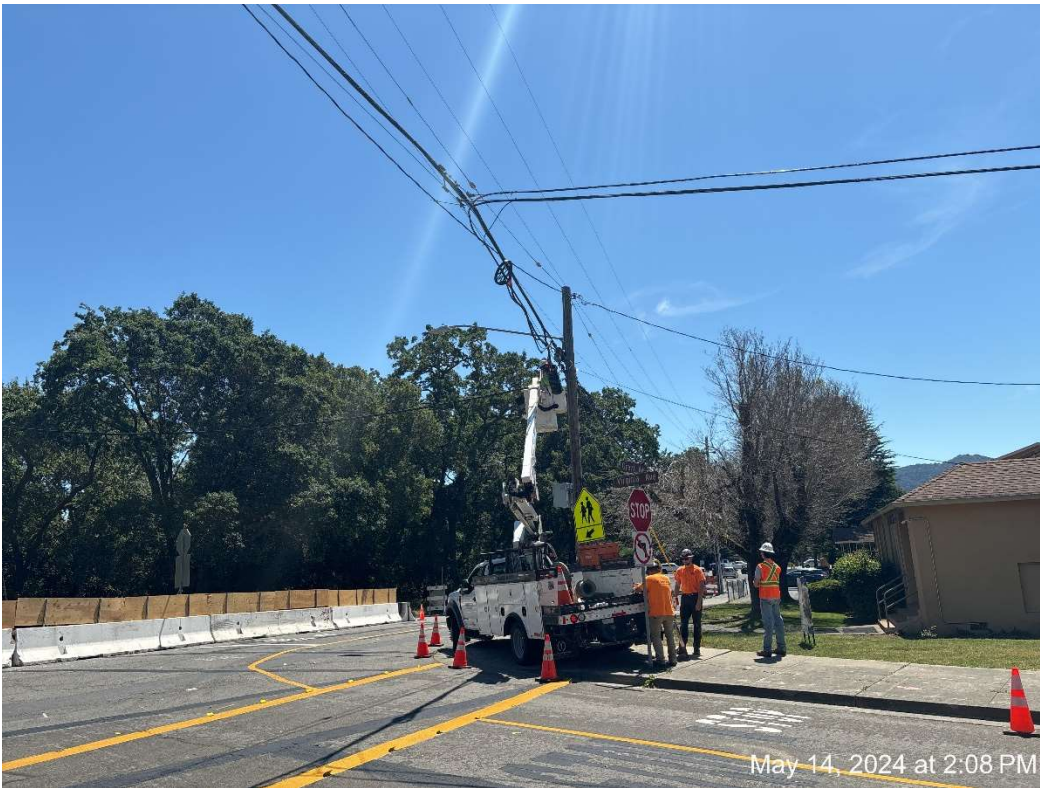
Figure 4 – Frontier Relocating OH Communication Line.
