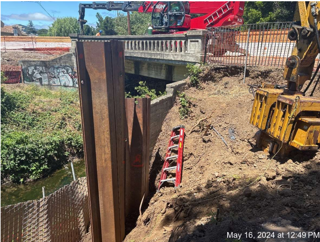
Figure 6 – Minerva installing Abutment 2 Sheetpile Shoring.
