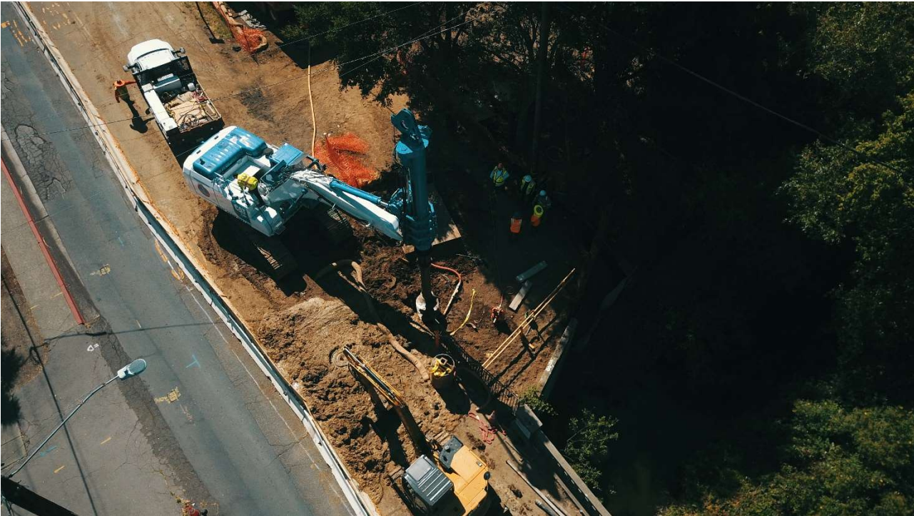
Figure 16 – Drone Picture of Drilling at Abutment 2.
