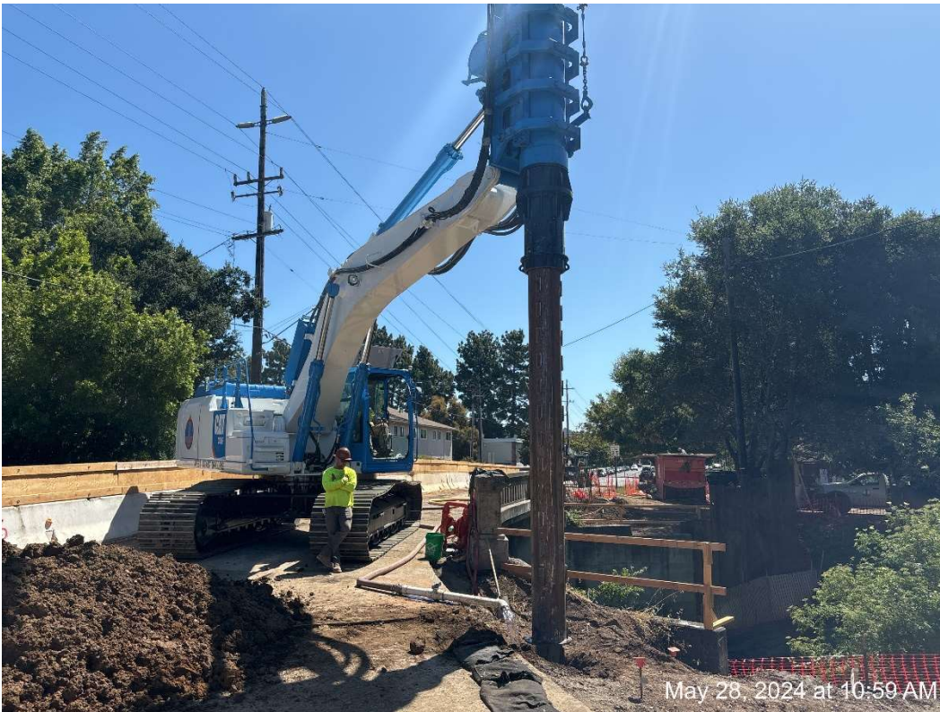
Figure 13 – West Coast Drilling continuing drilling the CIDH Pile.
