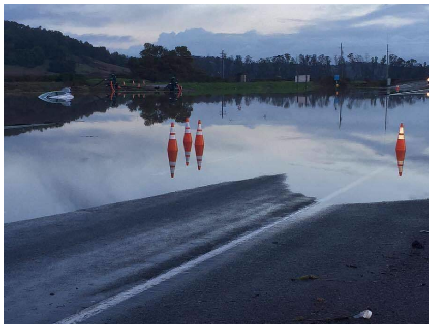
Figure 37: SR 37 Flooding in Novato - 2017 Source: The Santa Rosa Press Democrat
