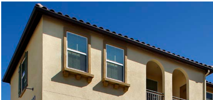
Window Frame/Trim Example: Composite Frame/Stucco Trim
