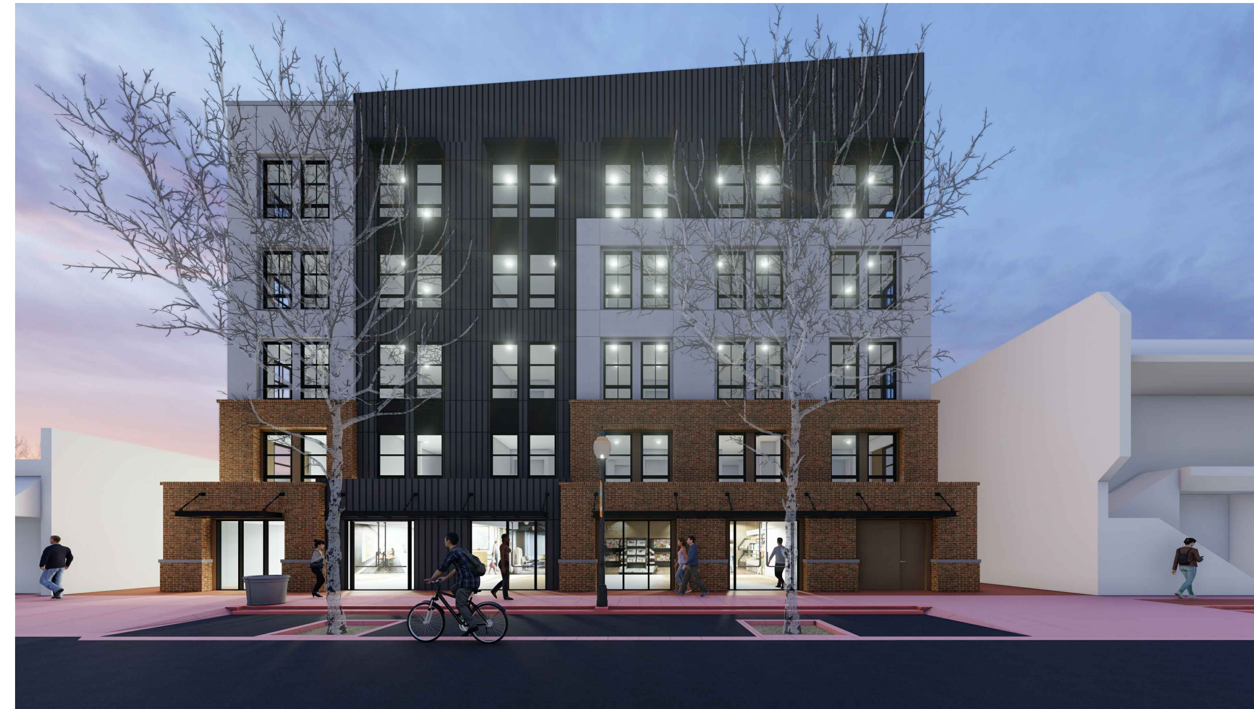
SOUTH ELEVATION VIEW FROM GRANT STREET 2
