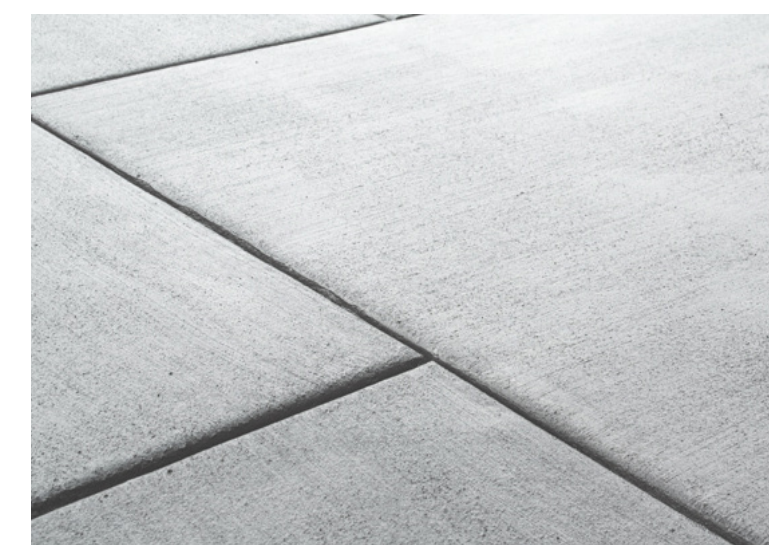
Concrete Walkways & Curbs
