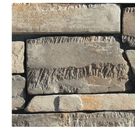
Stone Base at Pilaster
