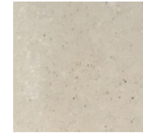
Precast at Pilaster
