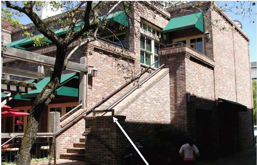
stairway adjacent to paseo is appropriately enclosed and trimmed with material (brick) consistent with the building
