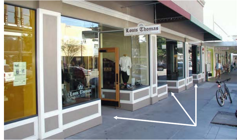
three remodeled storefronts due to fire retain composition and detailing of the original storefront
