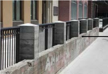
wall articulated with posts and metal railing
