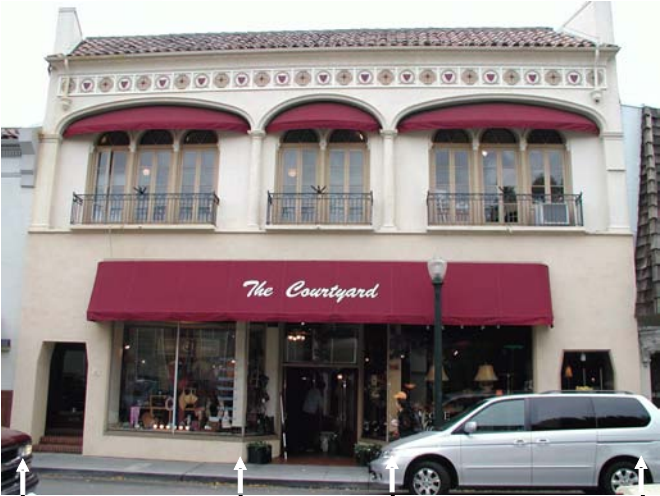
rhythm of ground floor modules is complemented through the balance and design of 2 nd story elements (french doors & balconies, decorated frieze, roof etc).
