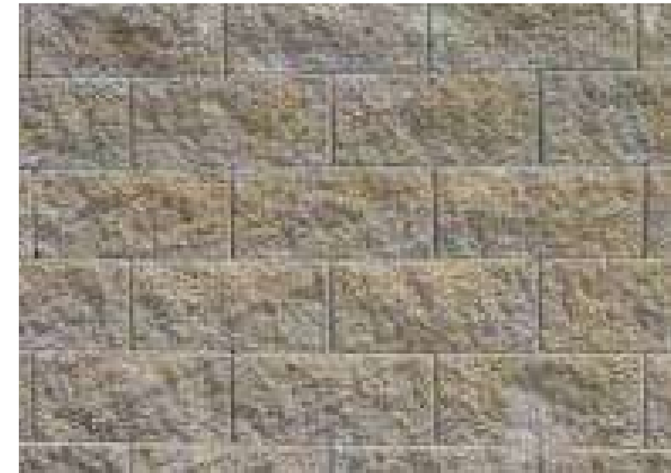
CMU RETAINING WALL
