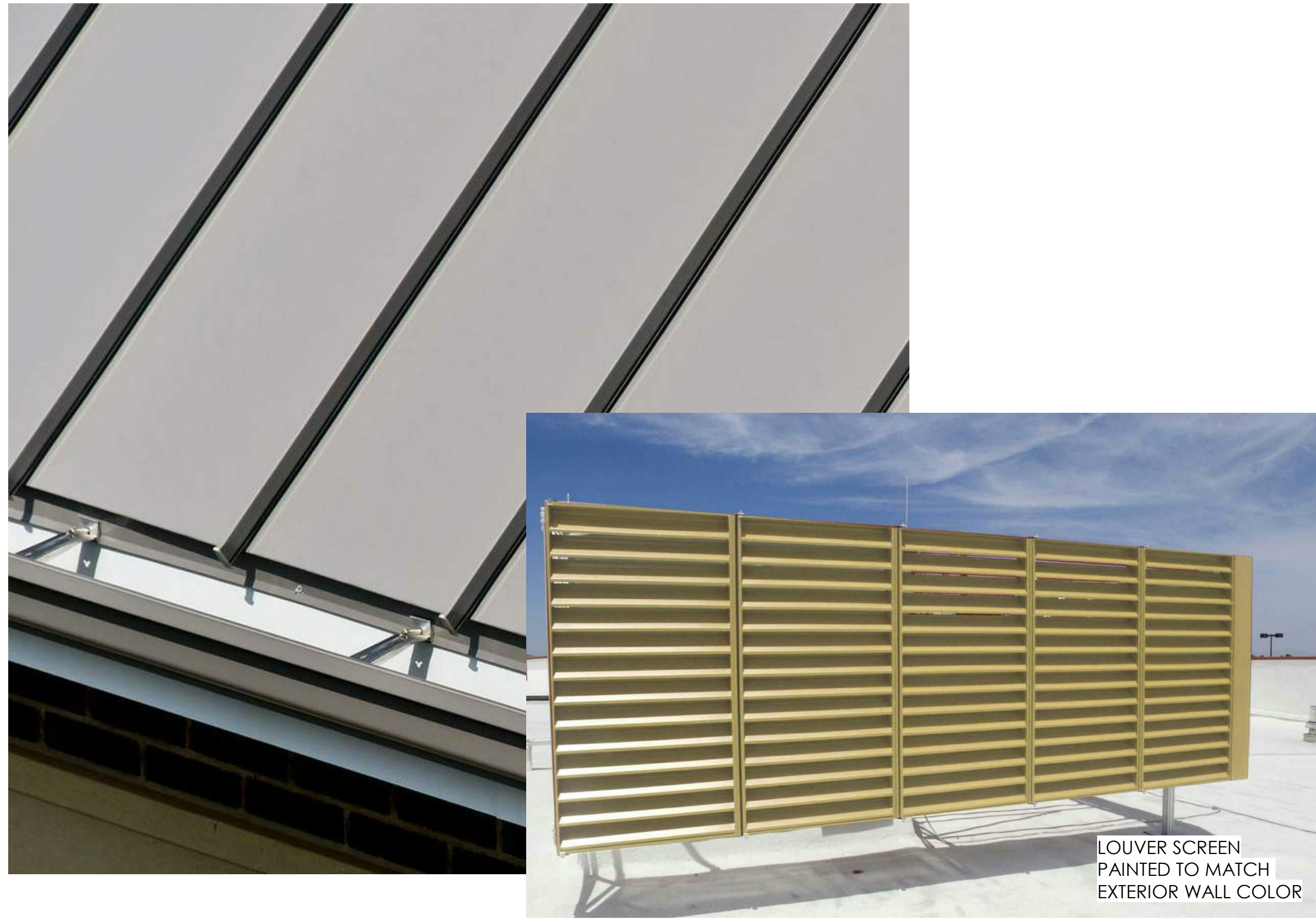
STANDING SEAM METAL ROOFING
