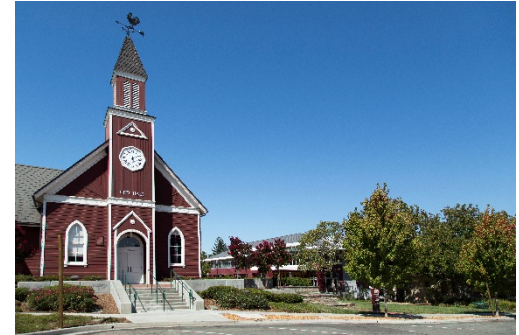
City Hall (former 1 st Presbyterian Church) Built 1896
