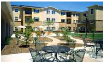
Livermore Independent Living Apartments Phase I
