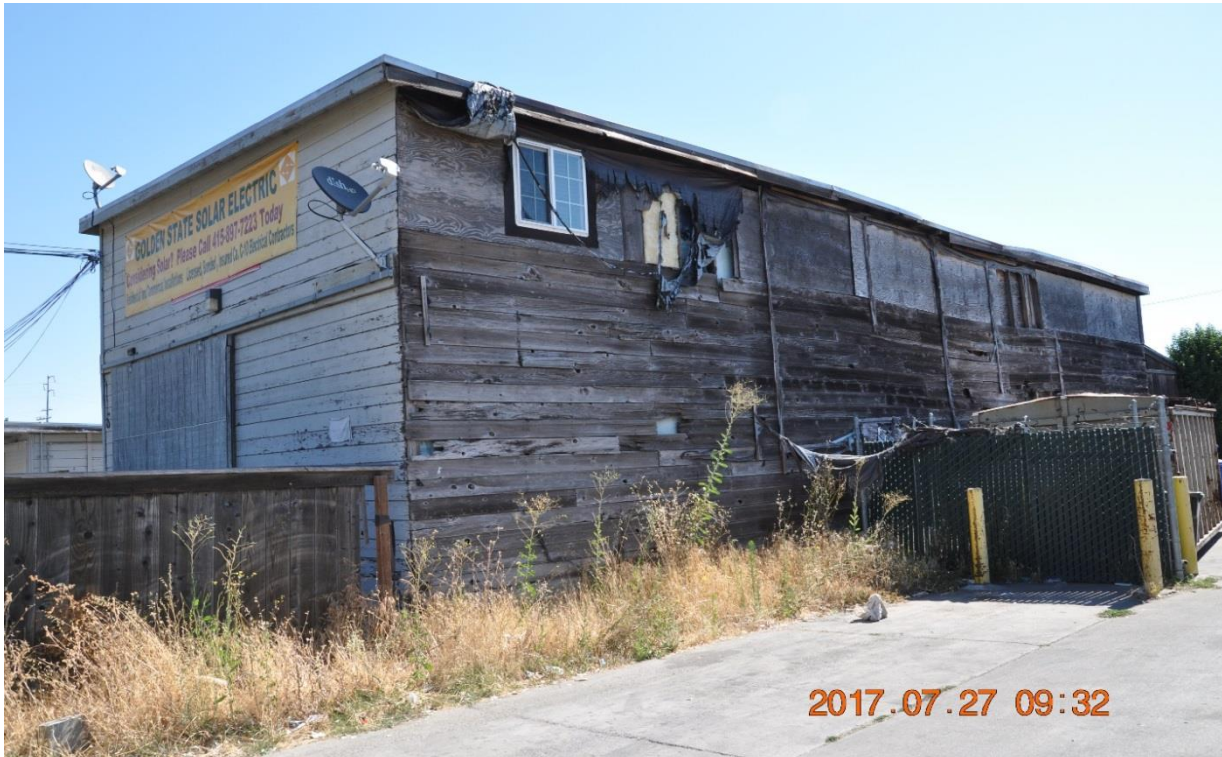
Photo 4: Project site southerly building (street view) (Building "B" on Photo 2)
