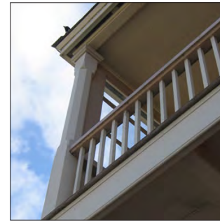
Typical wood-framed balcony/porch
