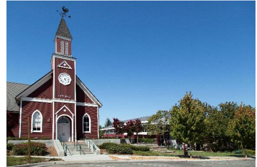
City Hall (former 1 st Presbyterian Church) Built 1896
