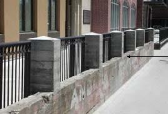
wall articulated with posts and metal railing
