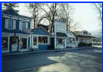
15 - Western Facade Type
