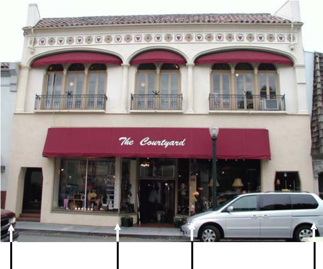
rhythm of ground floor modules is complemented through the balance and design of 2 nd story elements (french doors & balconies, decorated frieze, roof etc).
