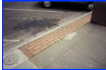
32 - Sidewalk Pavers with Utility Inset
