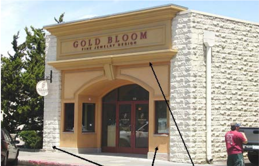
complementary but contrasting materials (stone, stucco and smooth wood trim) provide a distinctive, attractive finish to a façade
