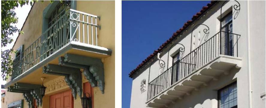
↑ well proportioned and detailed balconies ↑
