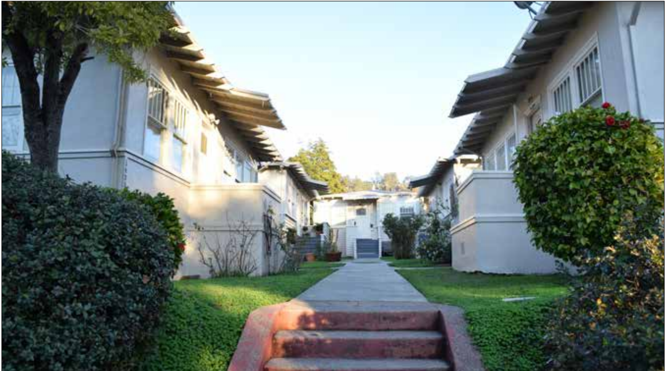
Five-building, one-story Cottage Court with stoop frontages along court leading to entries.
