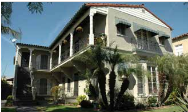
Two-story Multiplex Small with front yard and common open space along side.
