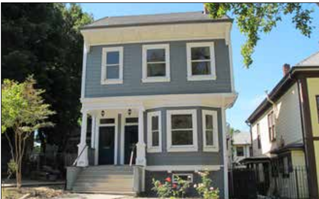
Two-story Duplex with stoop frontage.
