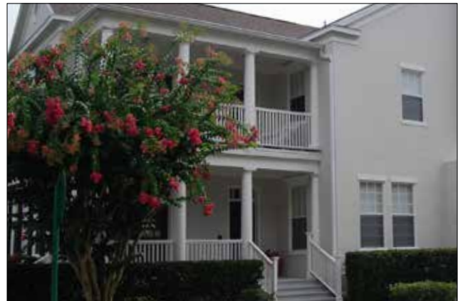
2-story engaged porch with its long side fronting the street.
