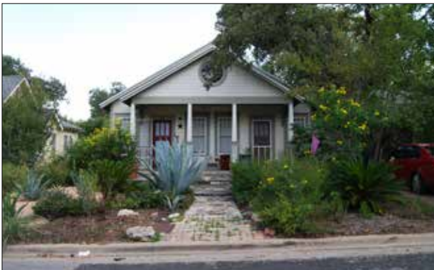
1½-story Duplex with both units accessed from the projecting porch.
