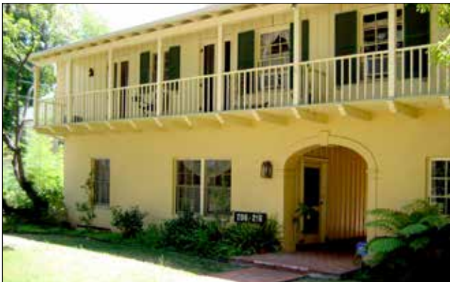
Courtyard passage from front yard to courtyard with ground floor windows and upper story balcony units facing the street.
