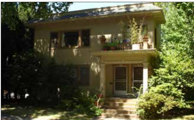
Two-story Duplex with stacked units and paired entries in projecting porch.
