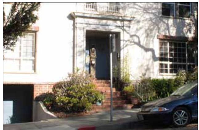
Stoop leading to prominent side street entry and visually enhanced by landscaping.
