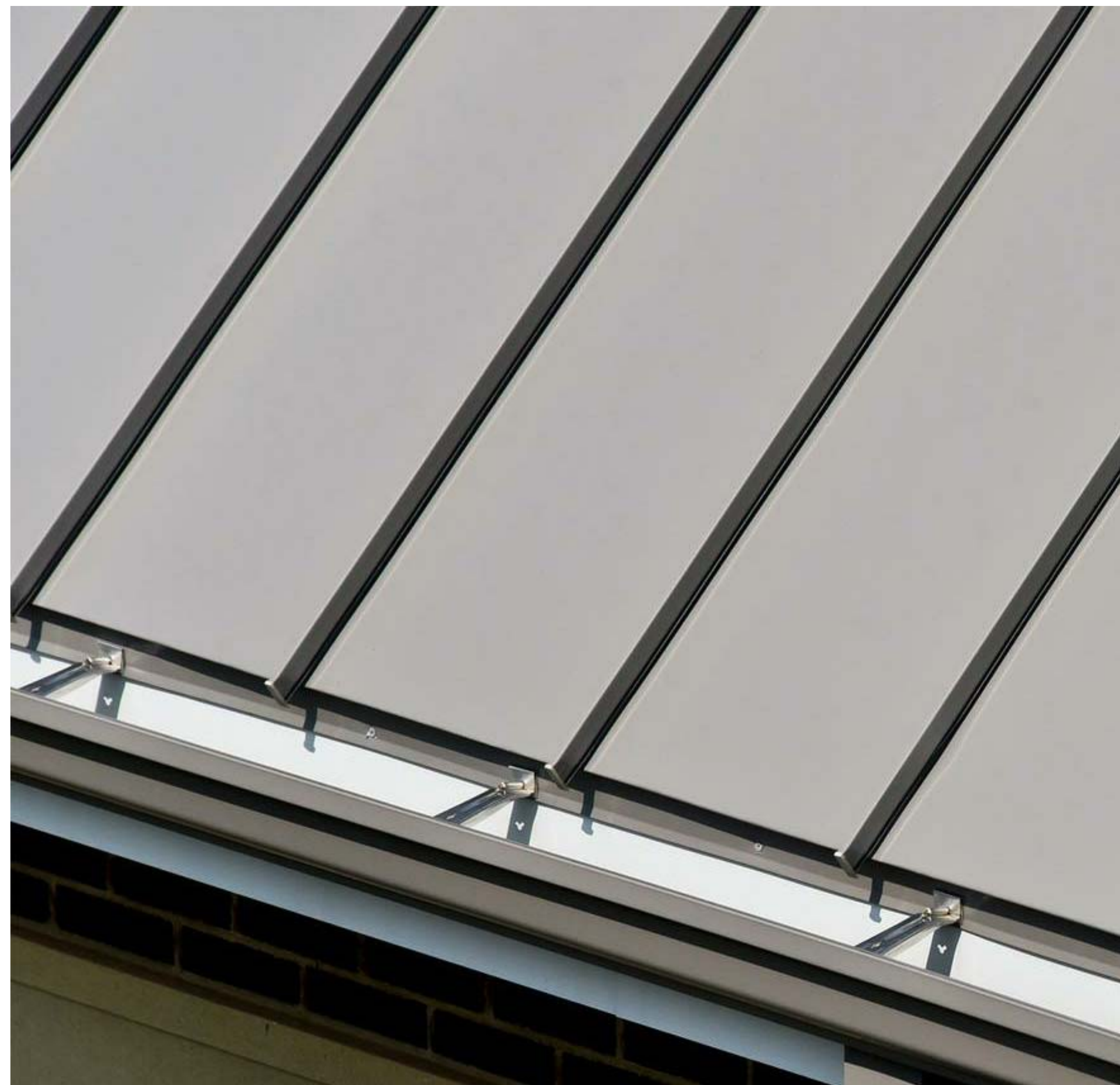
STANDING SEAM METAL ROOFING
