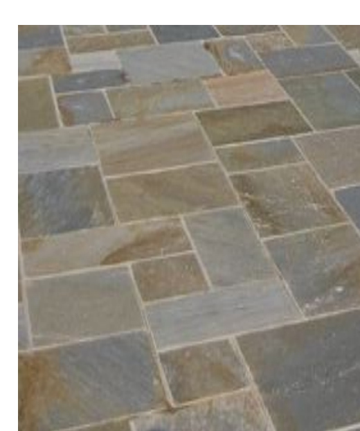
FRONT ENTRY WALKWAY - SLATE TILES
