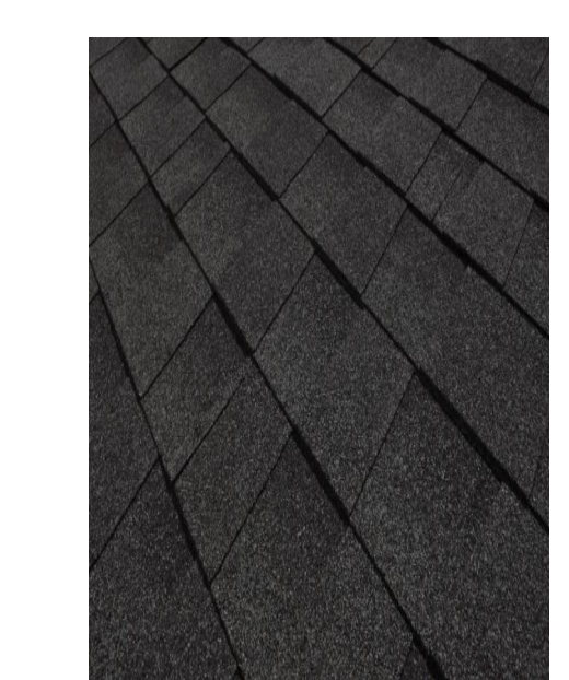
ROOF - ASPHALT SHINGLE ROOF
