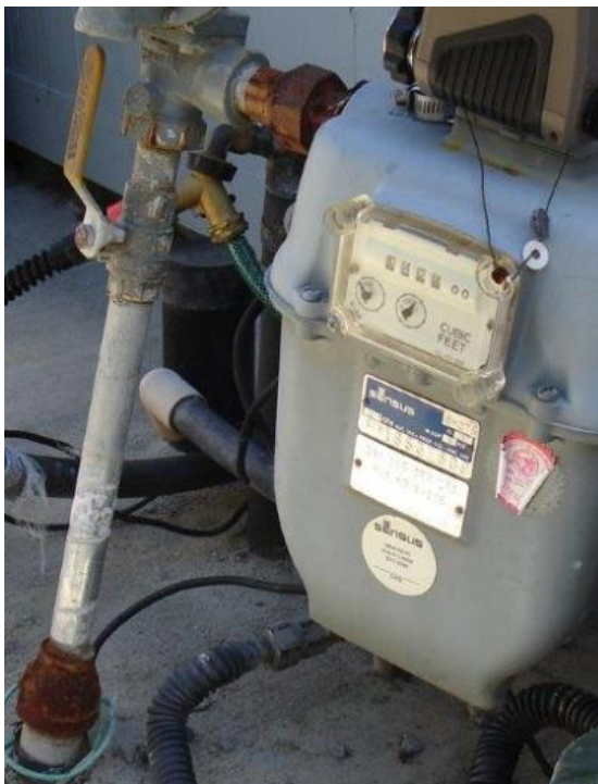
#3 -- NEW VALVE INSTALLED
