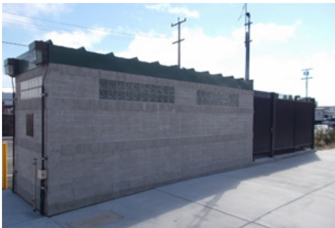
David Stier from Nute has been designing pump stations for over a decade. This photo is from the Sausalito Pump station.
