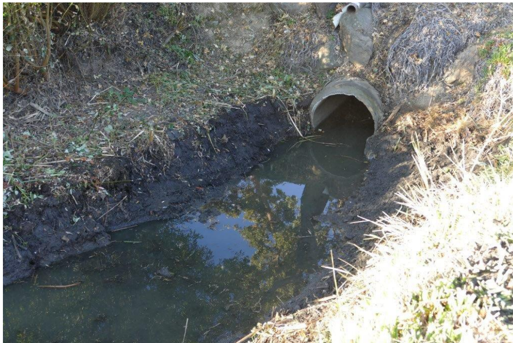
Looking West – End of Drain Pipe Cleared
