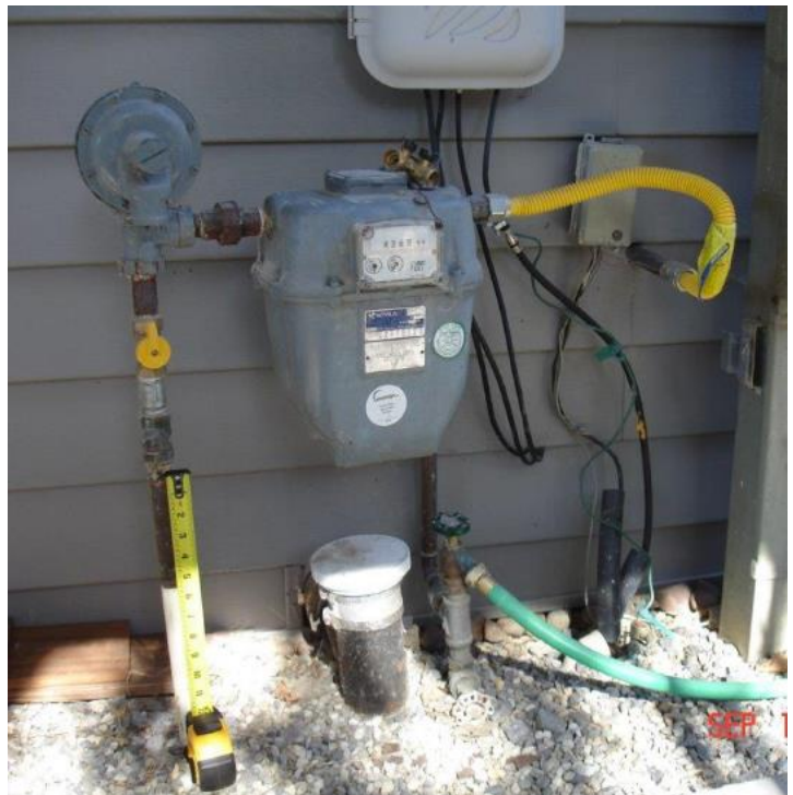
#4 -- NEW VALVE INSTALLED
