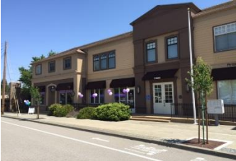
Umpqua Bank Building (999 Grant)
