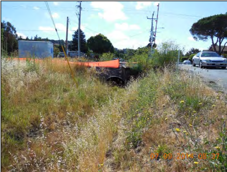
Olive Avenue Ditch looking east.
