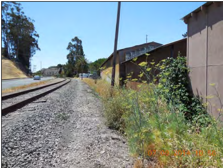
Railroad Ditch looking south towards Sweetzer Avenue – this portion of the ditch has wetland plants.
