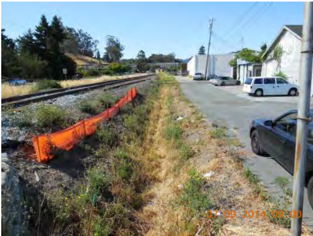
Figure 9. Railroad ditch looking south from Olive Avenue
