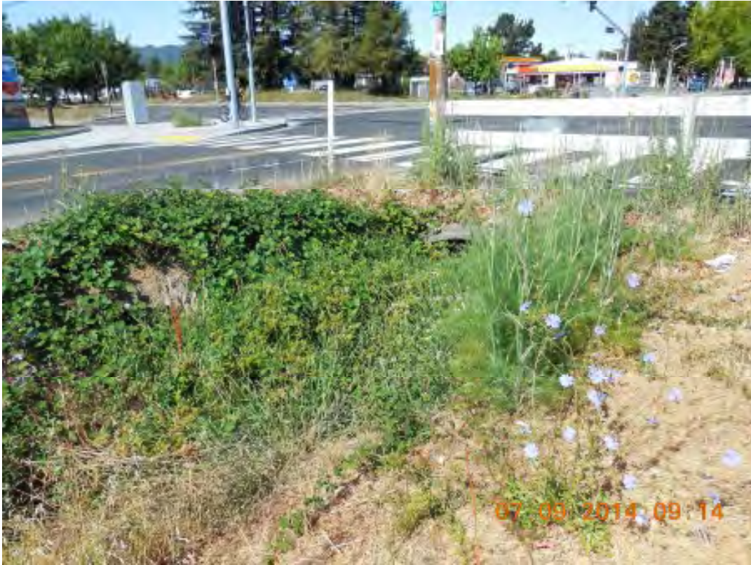
Figure 4. Culvert and drainage ditch at Olive and Redwood Avenues.
