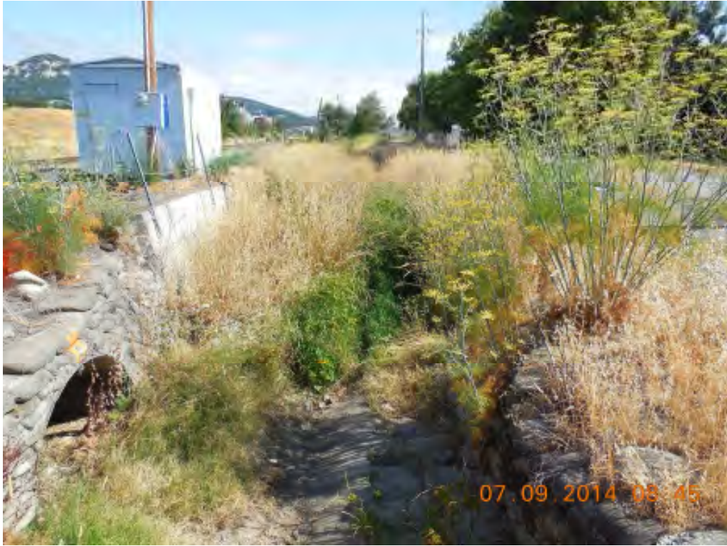
Figure 8. Bowl at Olive Avenue on east side of SMART railroad crossing.
