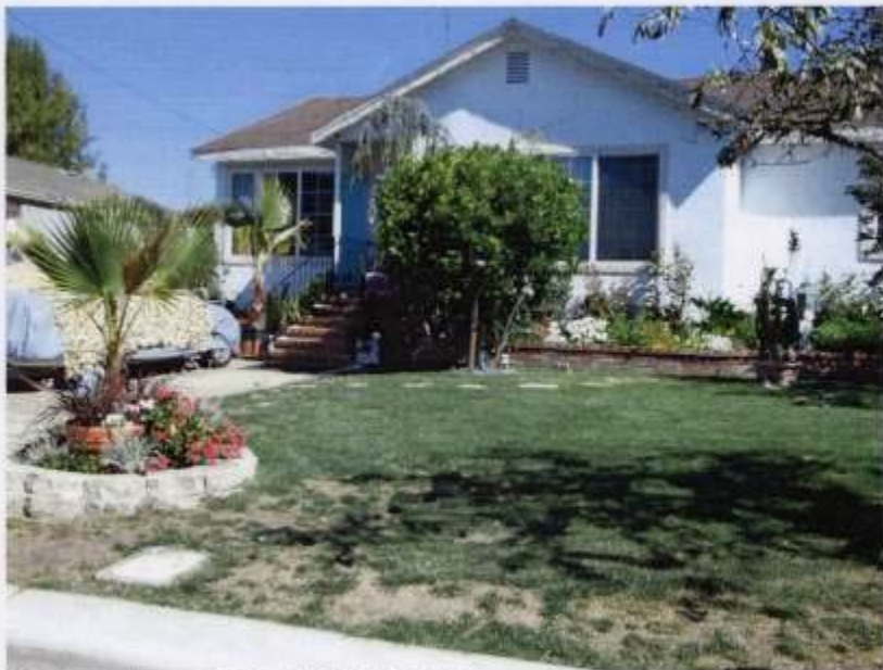
19 Joan Ave. APN. 140-141-01 Elevated Home Site #5
