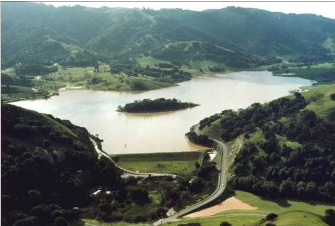
Novato Creek Dam
