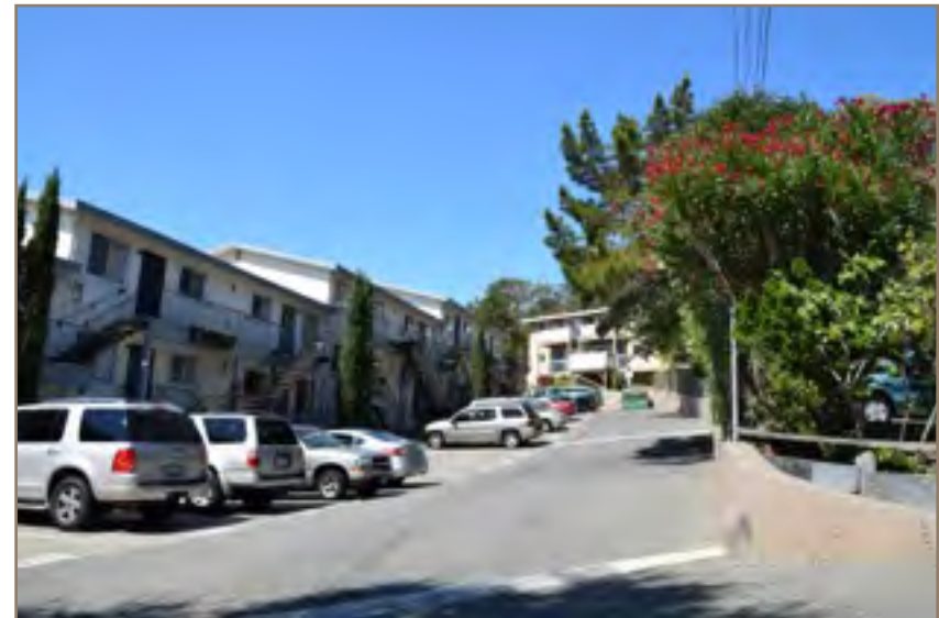
Parking dominates site
