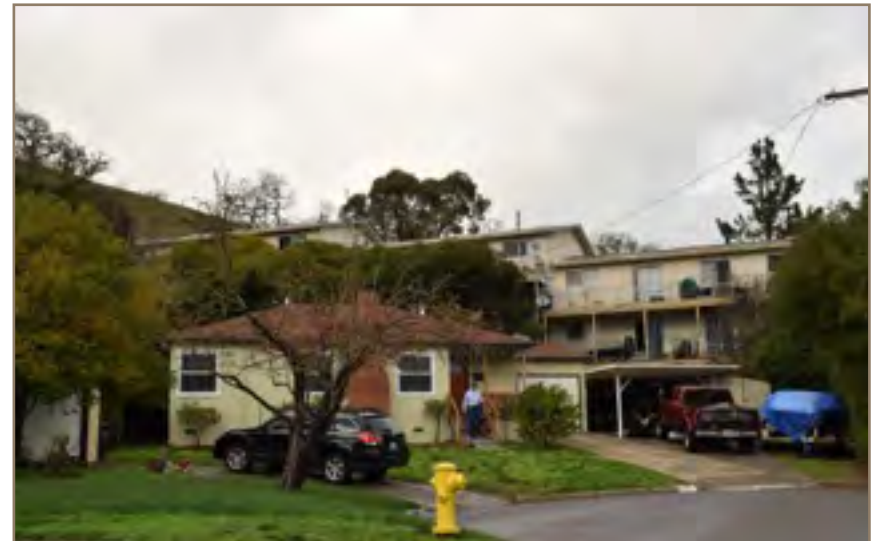
Incompatible building scales
