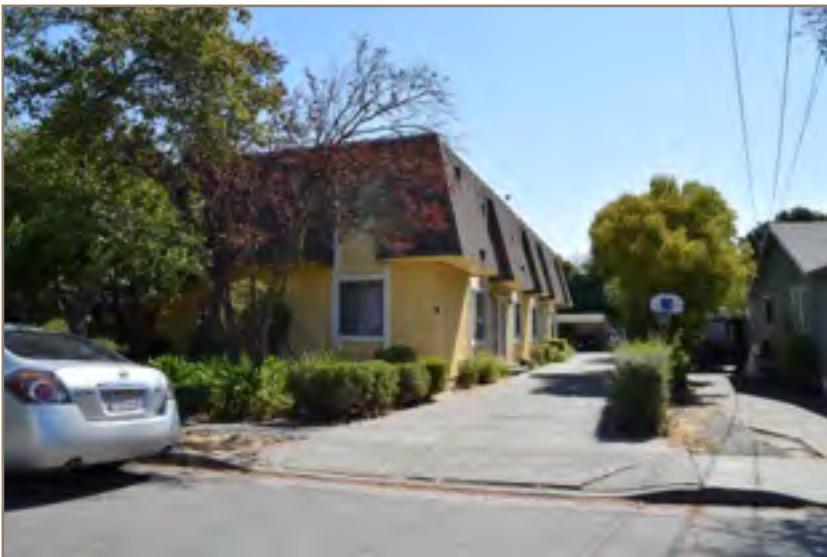
Mansard roof fails to reduce perception of building's height and bulk.
