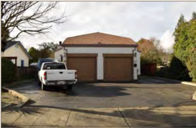
Garage doors and drives dominate fronts
