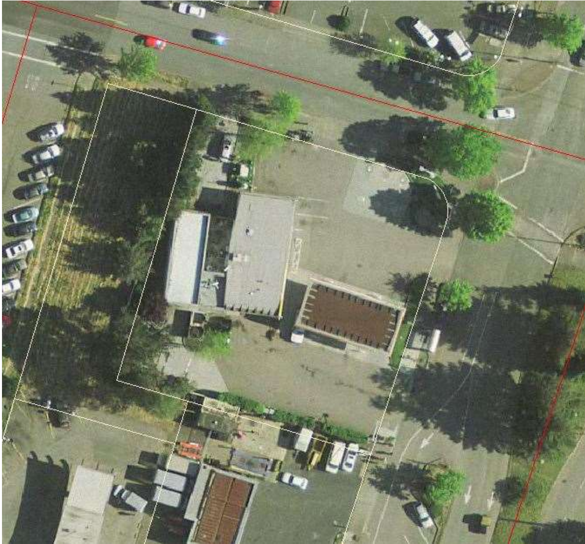
Existing site layout at 7473 Redwood Boulevard
